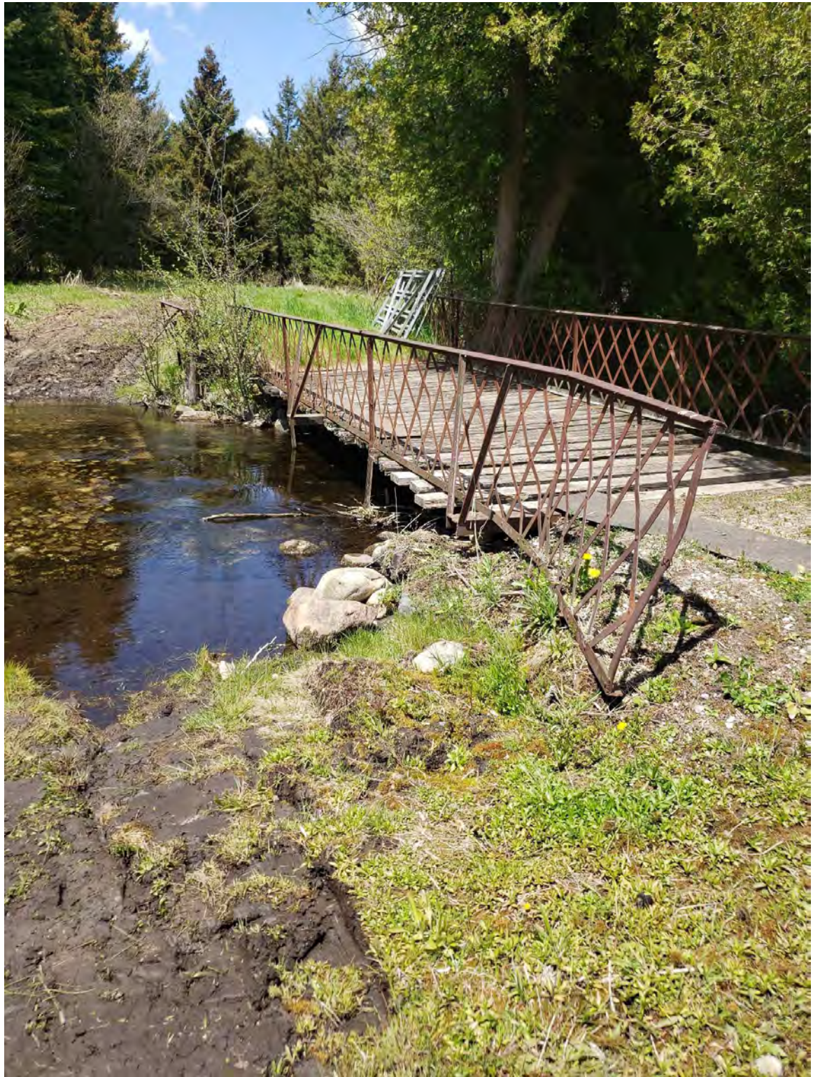
Tributary 1-1_ Bank Undercutting_structural damage-bridge__PS(5)_3.jpeg
