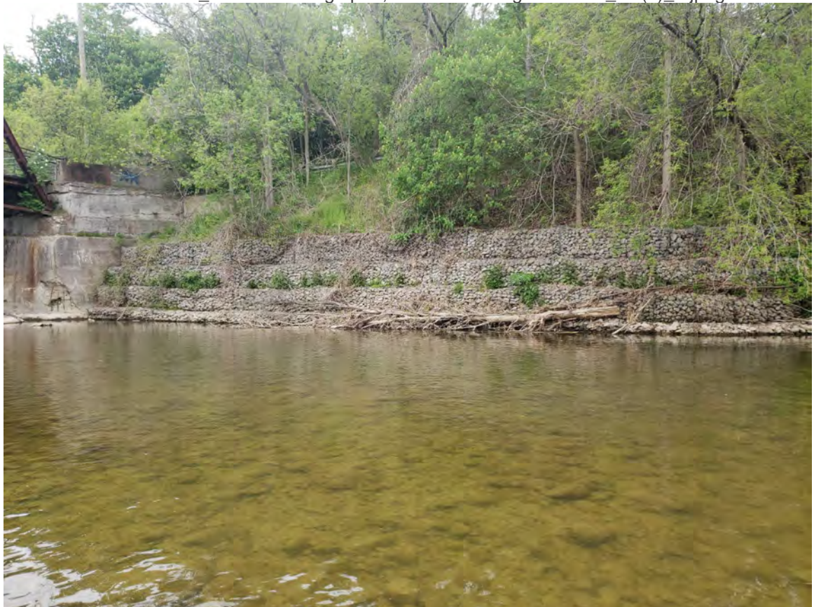
Nift River 4-4_concrete falling apart, tree debris on gabion wall_PS(3)_2.jpeg
