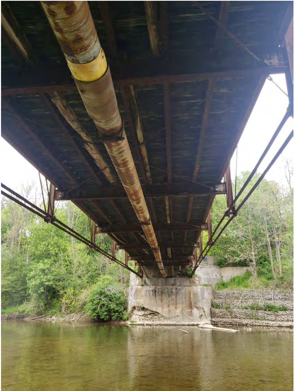
Nift River 4-4_concrete falling apart, tree debris on gabion wall_PS(3)_4.jpeg
