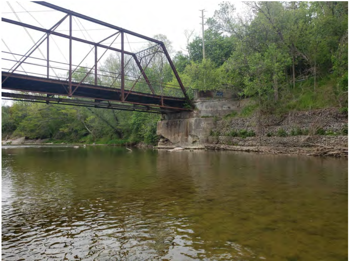
Nift River 4-4_concrete falling apart, tree debris on gabion wall_PS(3)_1.jpeg
