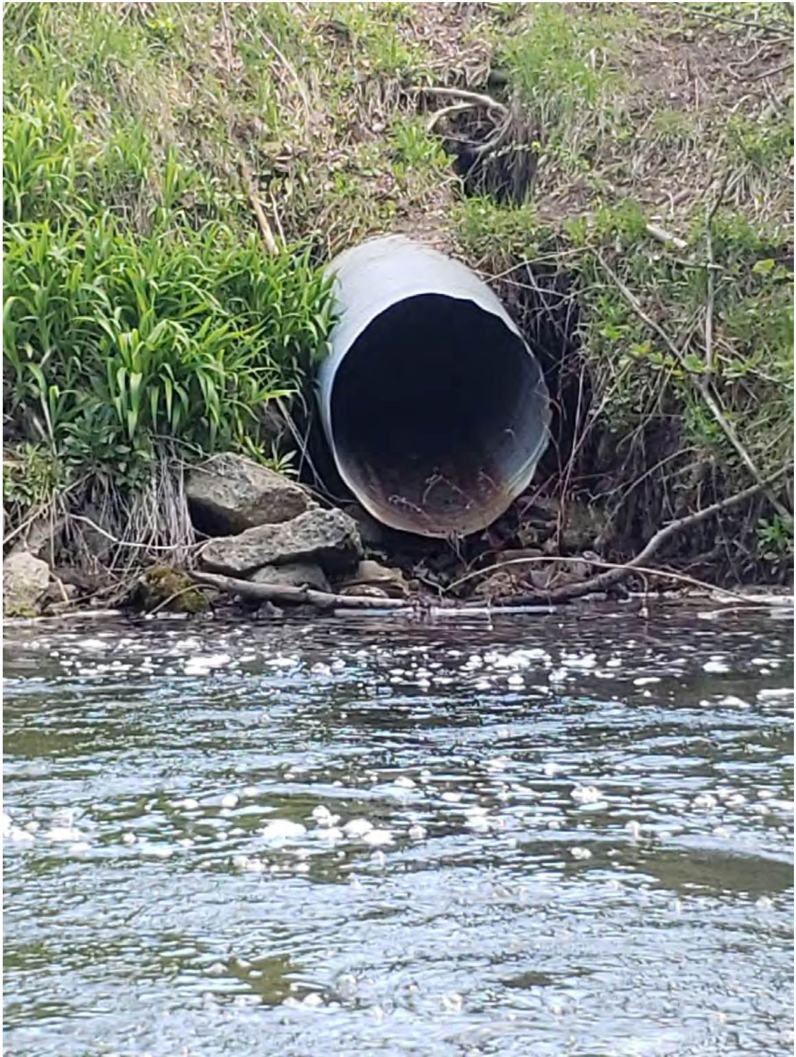
Tributary 1-1_Perched Culvert_PS(1)_2.jpeg
