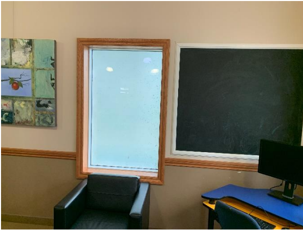
Photograph No. 7 Failed glazing seal in IGU
