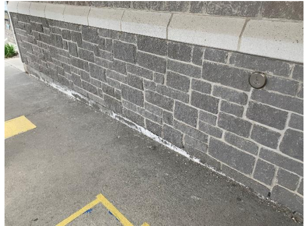
Photograph No. 4 - Minor foundation deterioration
