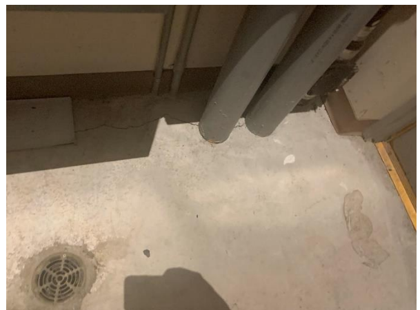
Photograph No. 24 Floor crack in mechanical room
