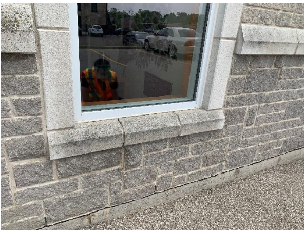
Photograph No. 5 Mortar joint erosion at window sill
