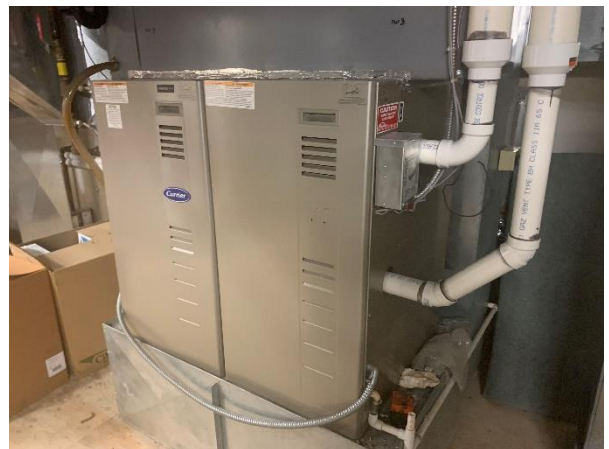
Photograph No. 18 Forced air furnace.
