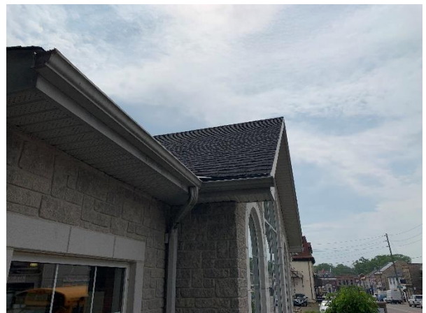
Photograph No. 12 New asphalt shingles
