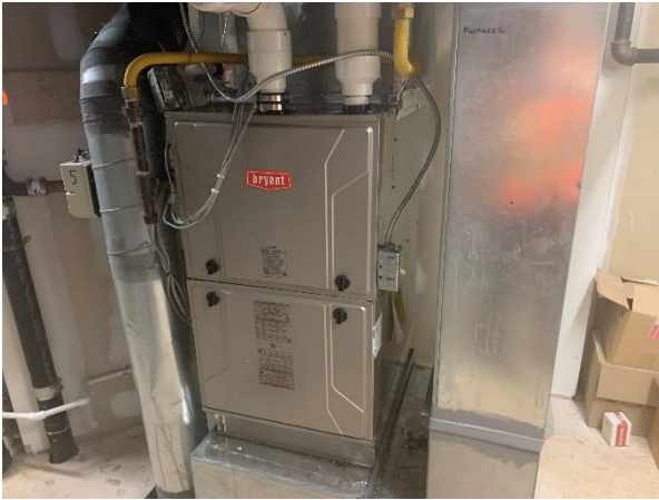
Photograph No. 19 New forced air furnace
