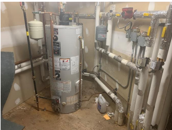
Photograph No. 17 Domestic water tank heater
