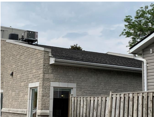
Photograph No. 11 Aged and curled asphalt shingles
