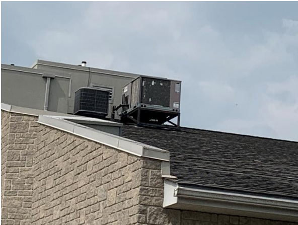
Photograph No. 21 Packaged rooftop HVAC unit and air conditioner
