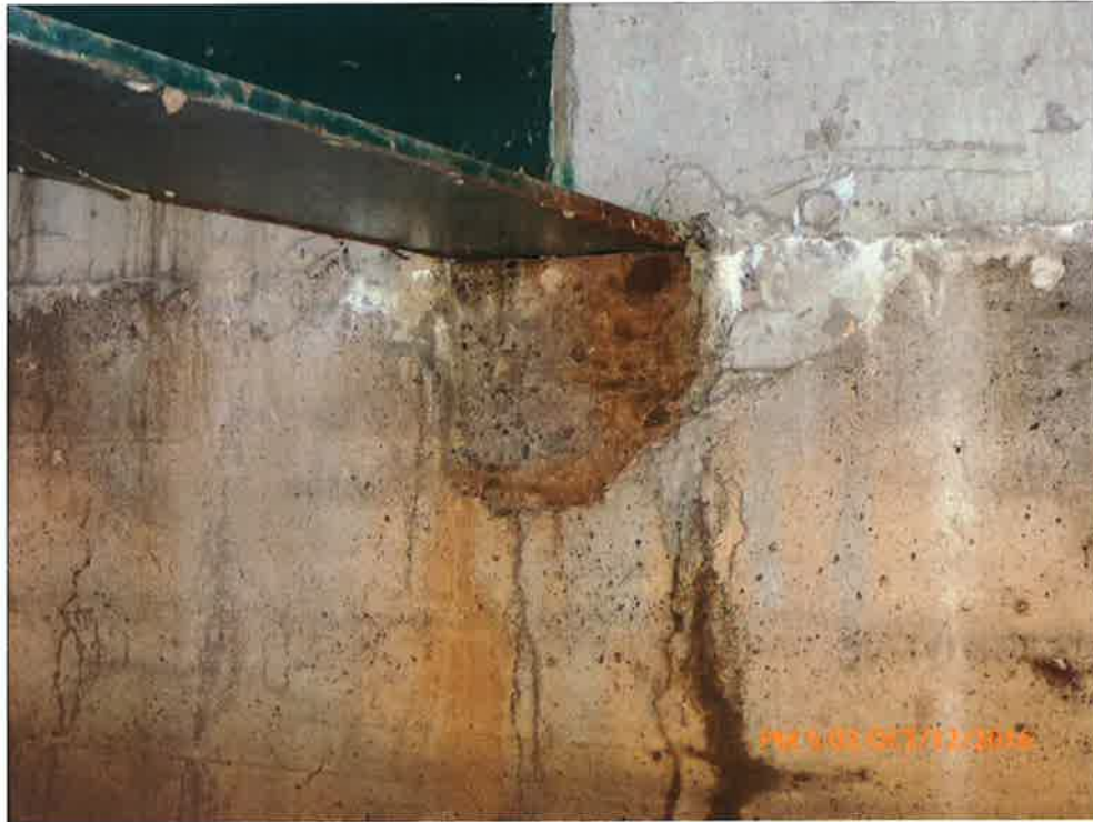
Light Spall on Abutment Below Girders
