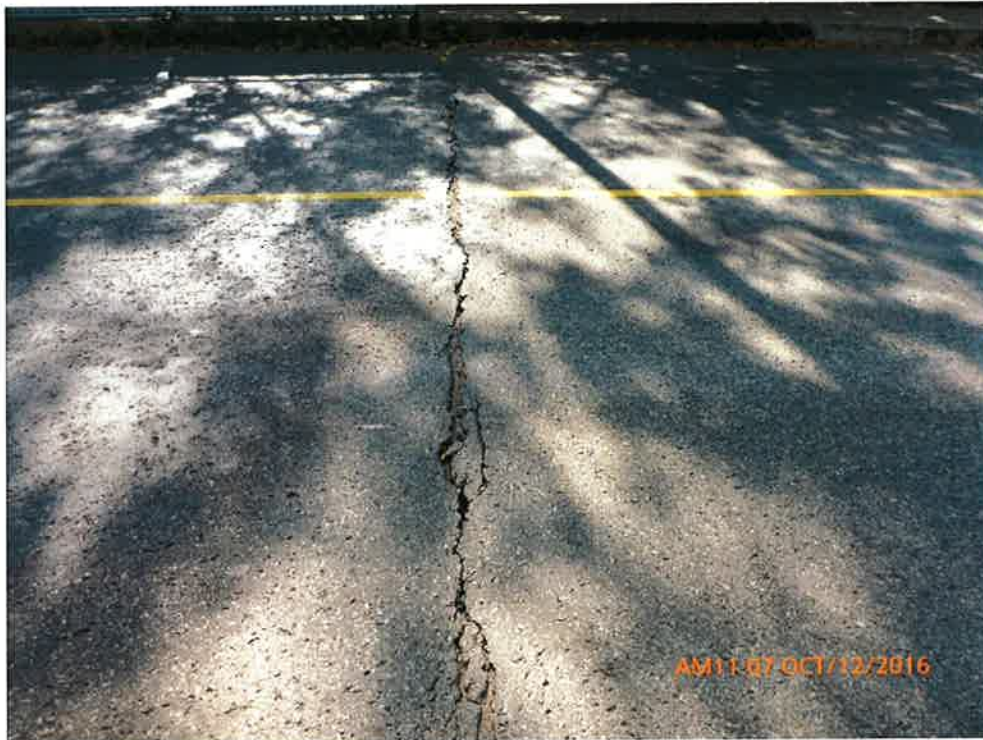
Wide Crack at End of Deck on Approach
