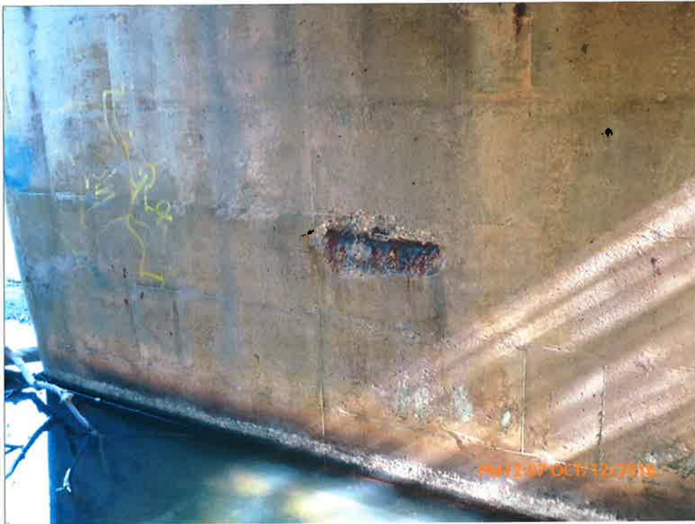
Severe Spall on Pier
