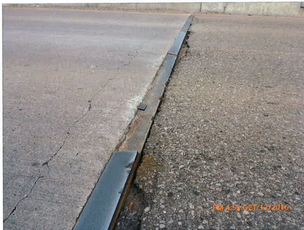
Missing Section of Armoring Angle
