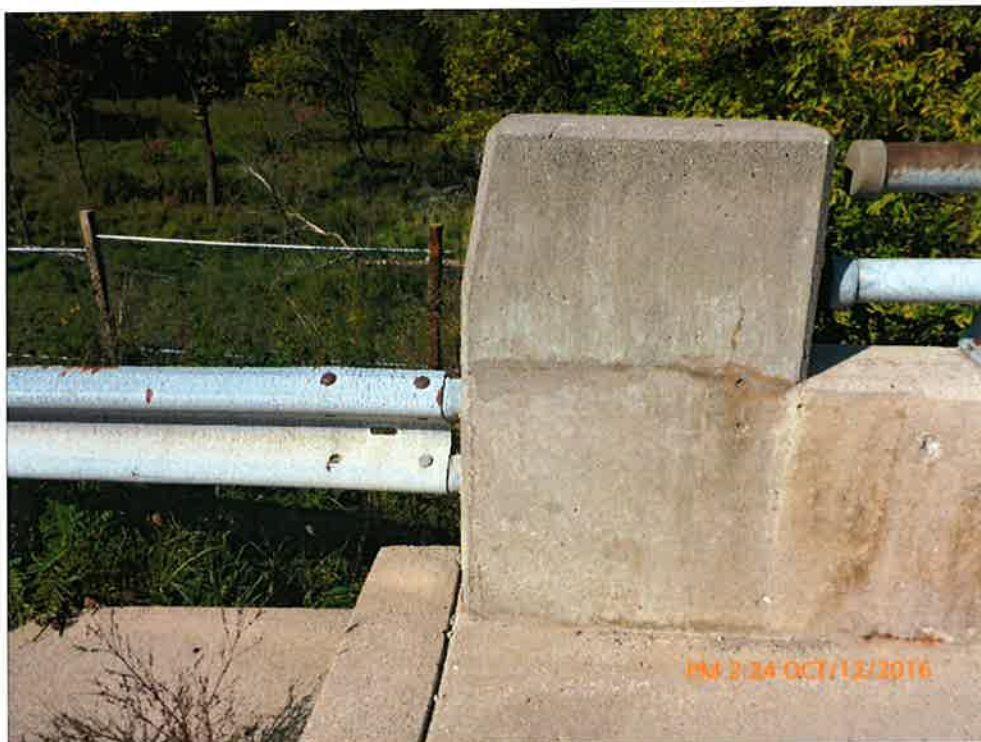
Below Standard Guiderail Connection
