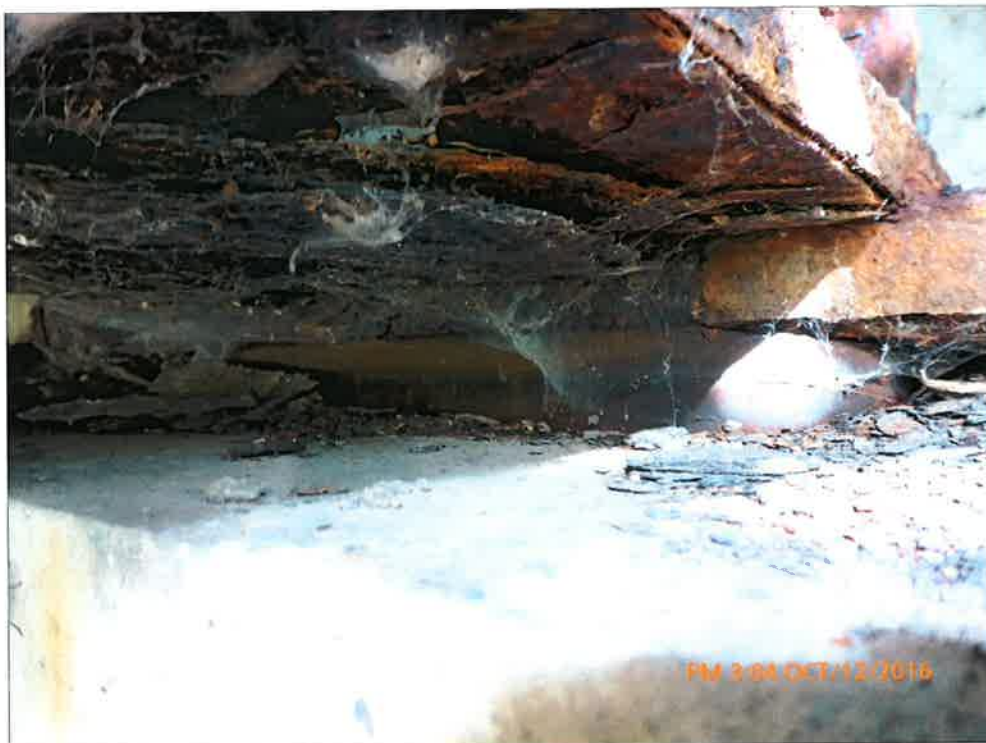
Severe Squashing of East Abutment Bearing
