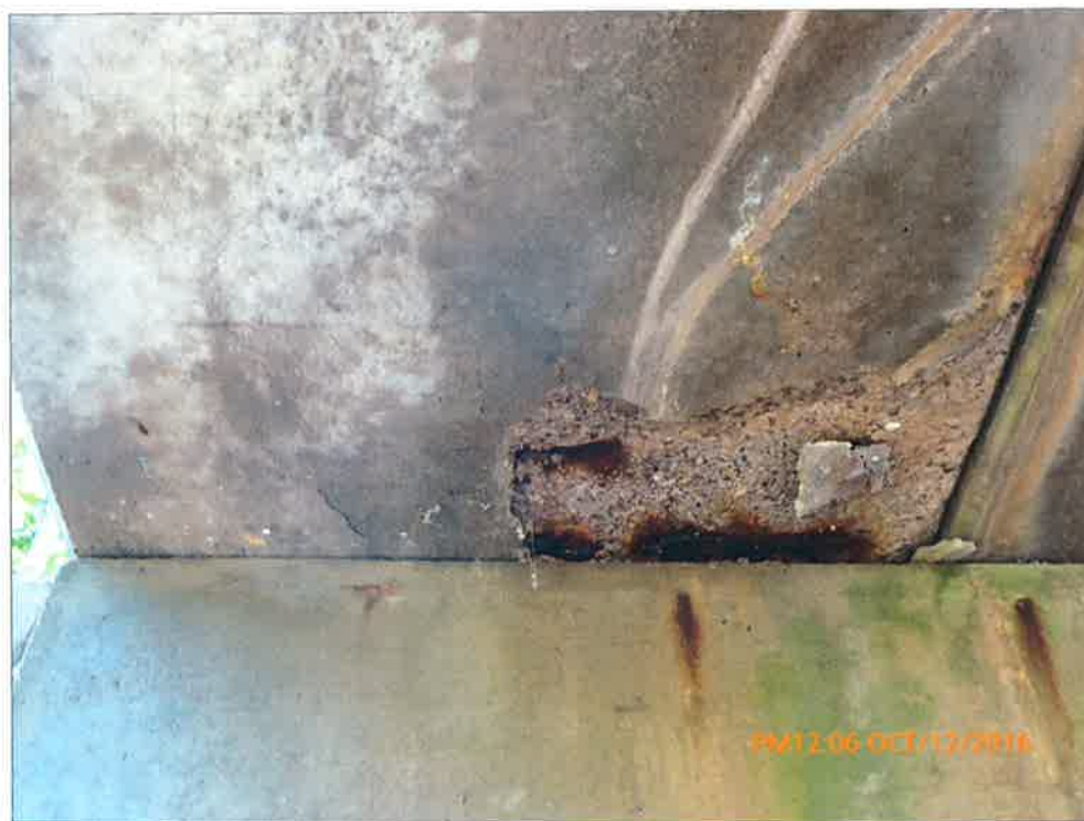
Severe Spall on Beam at End
