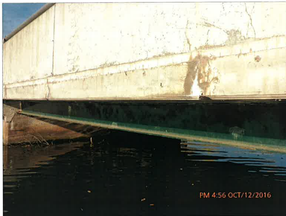
Narrow Stained Cracks on Exterior Soffit
