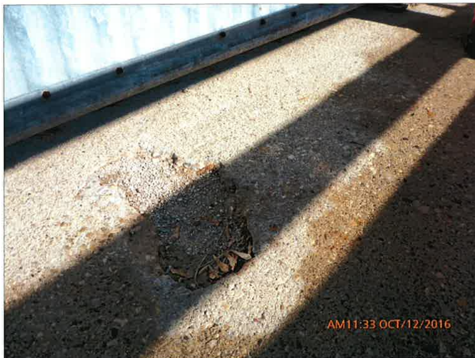
Severe Delamination on Sidewalk
