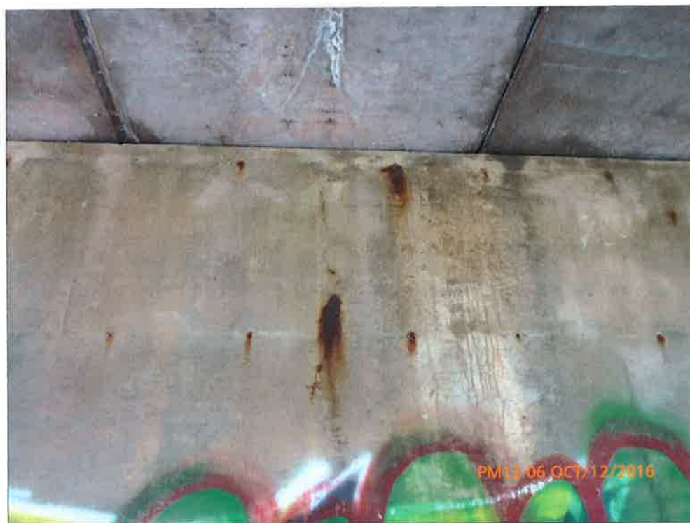
Rust Stains on Abutment Wall
