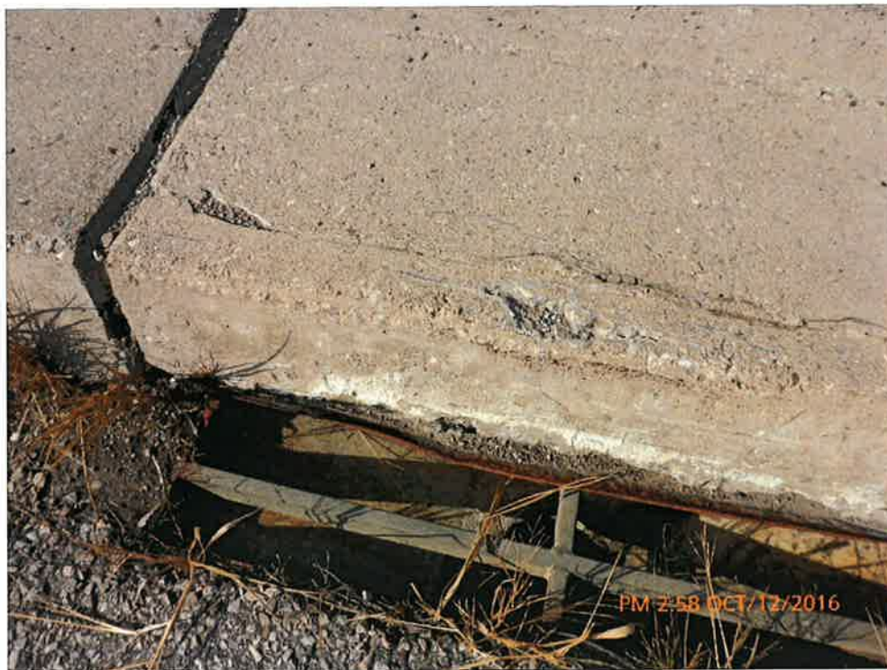
Delamination on Curb
