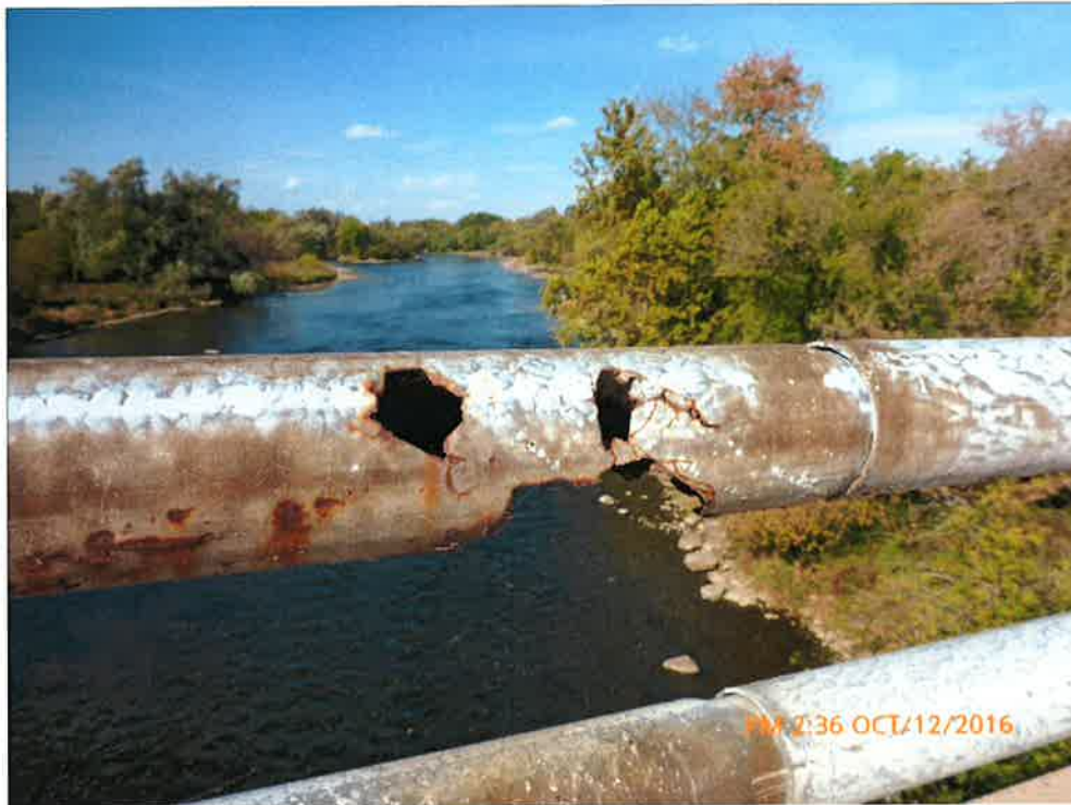
Severe Corrosion and Perforations on Handrail
