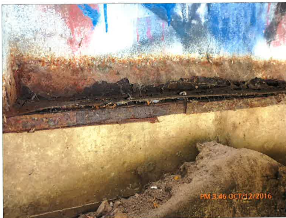
Medium Corrosion on End Diaphragm
