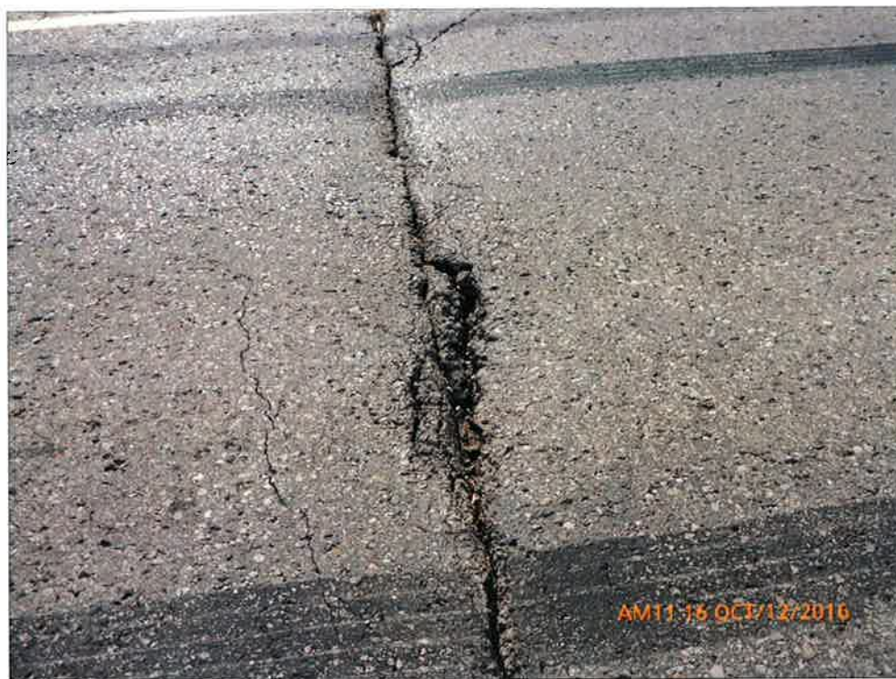
Localized Wide Cracks on Deck Wearing Surface
