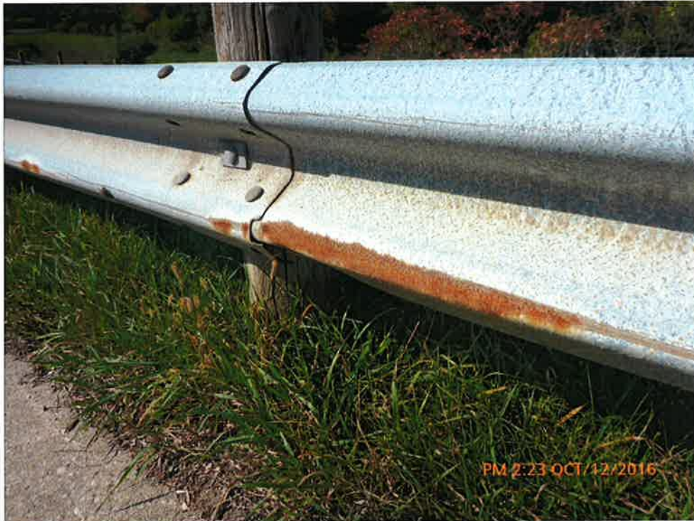
Minor Breakdown of Protective Coating
