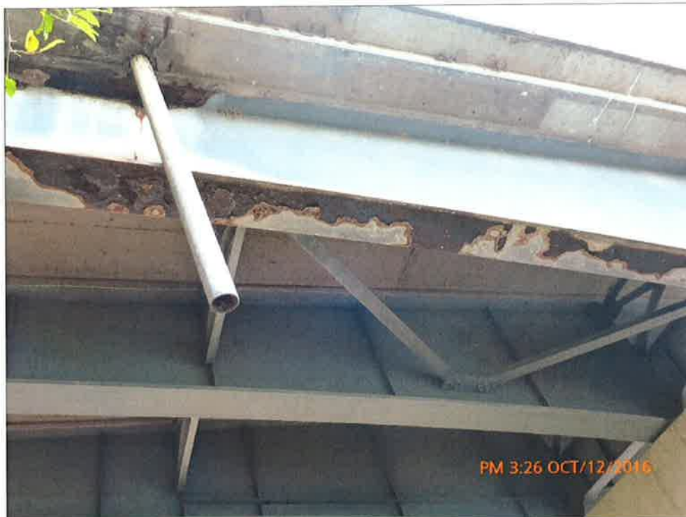
Breakdown of Protective Coating
