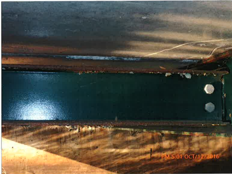
Light Corrosion on Diaphragm
