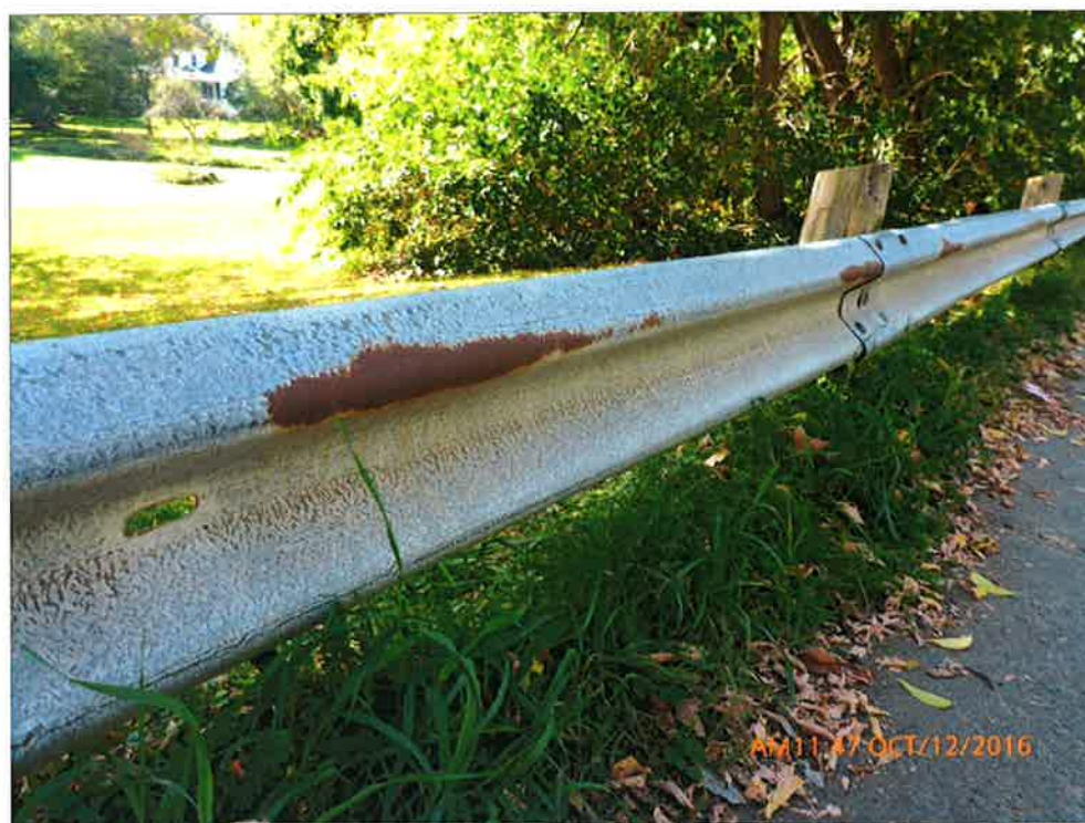
Localized Breakdown of Protective Coating on Approach Guiderail
