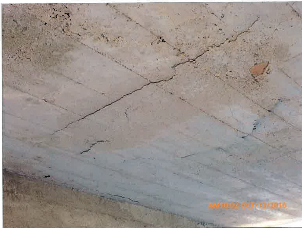
Severe Delamination on Interior Soffit
