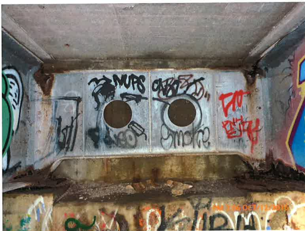
Typical End Diaphragm
