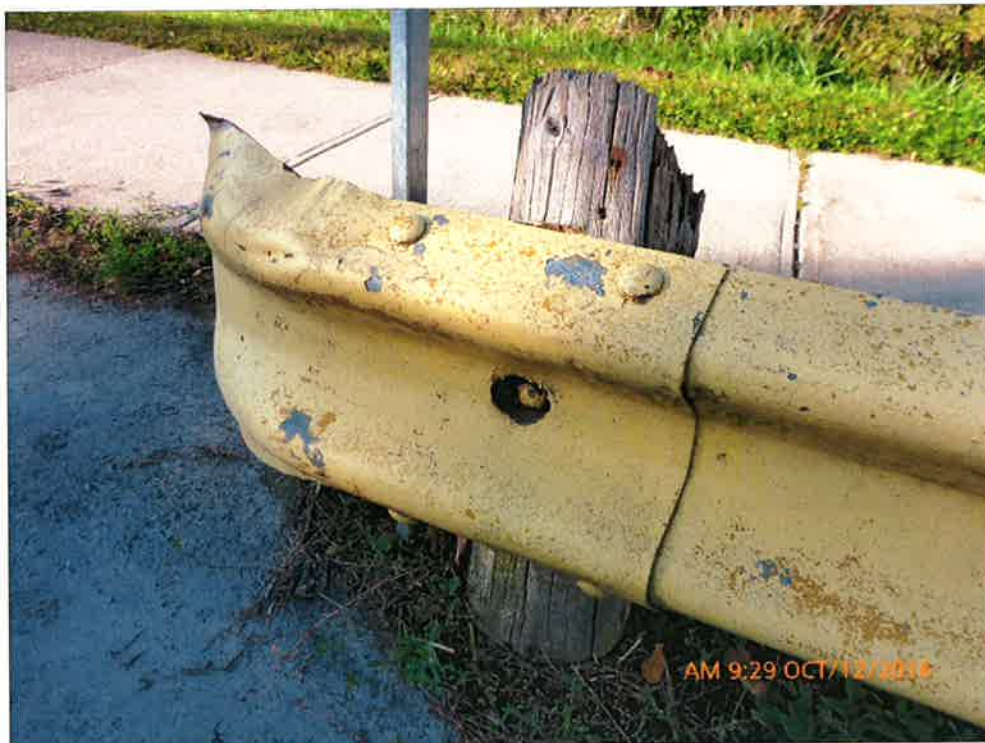
Guiderail Not Attached to Post
