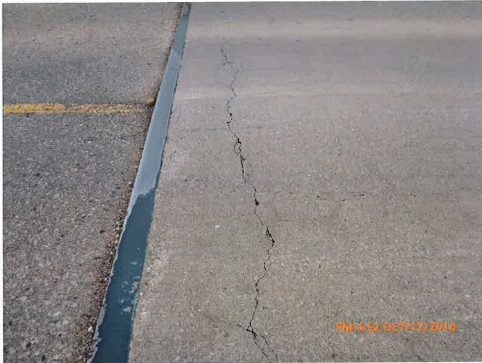
Wide Crack on Exposed Concrete Deck
