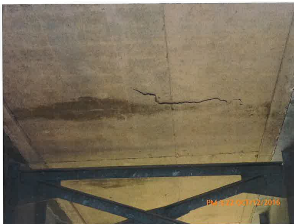
Delamination on Interior Soffit
