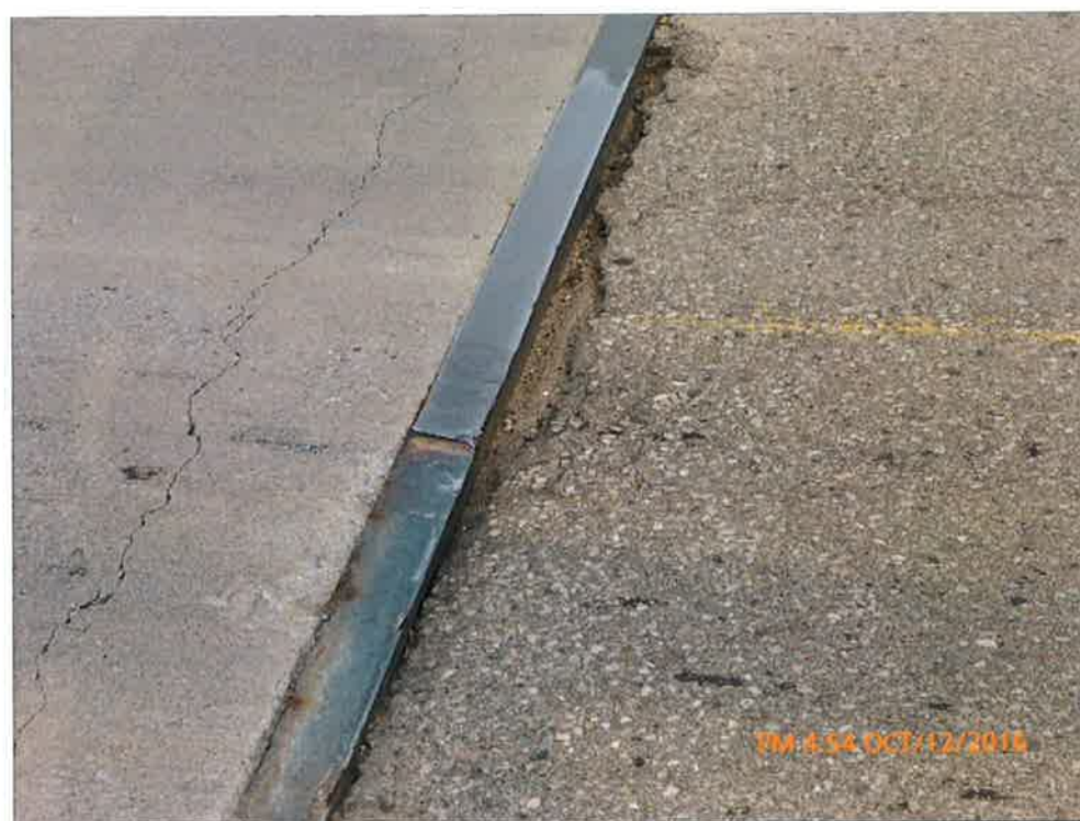
Pothole on Approach Wearing Surface
