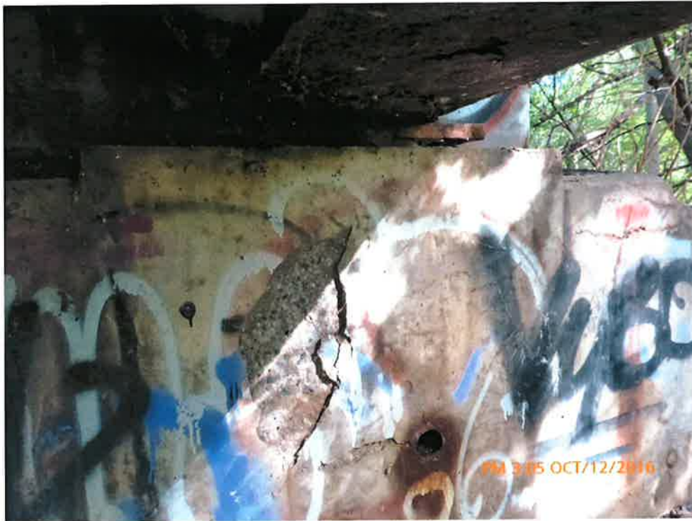
Delamination on Abutment Wall
