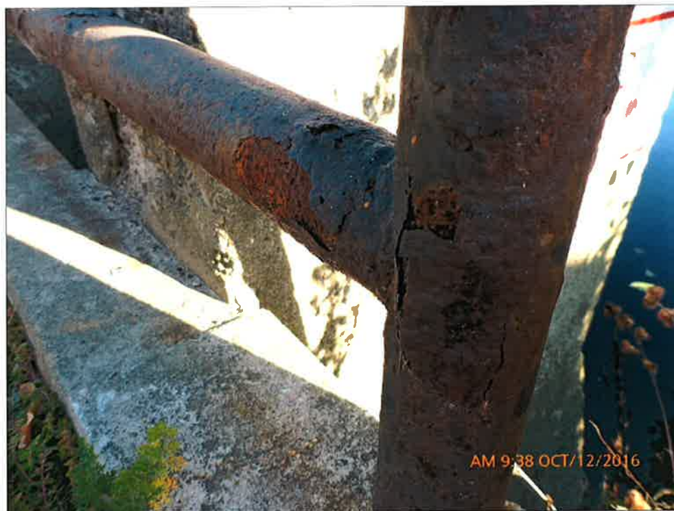
Flaking of Protective Coating on Handrail
