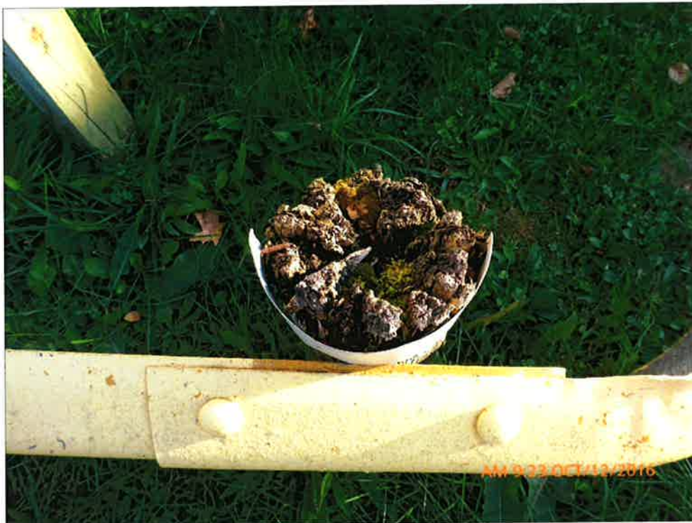
Severe Rot on Approach Guiderail Post
