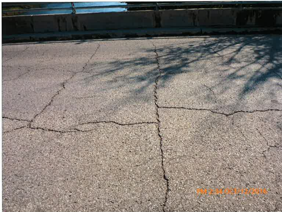
Wide Cracks on Deck Wearing Surface
