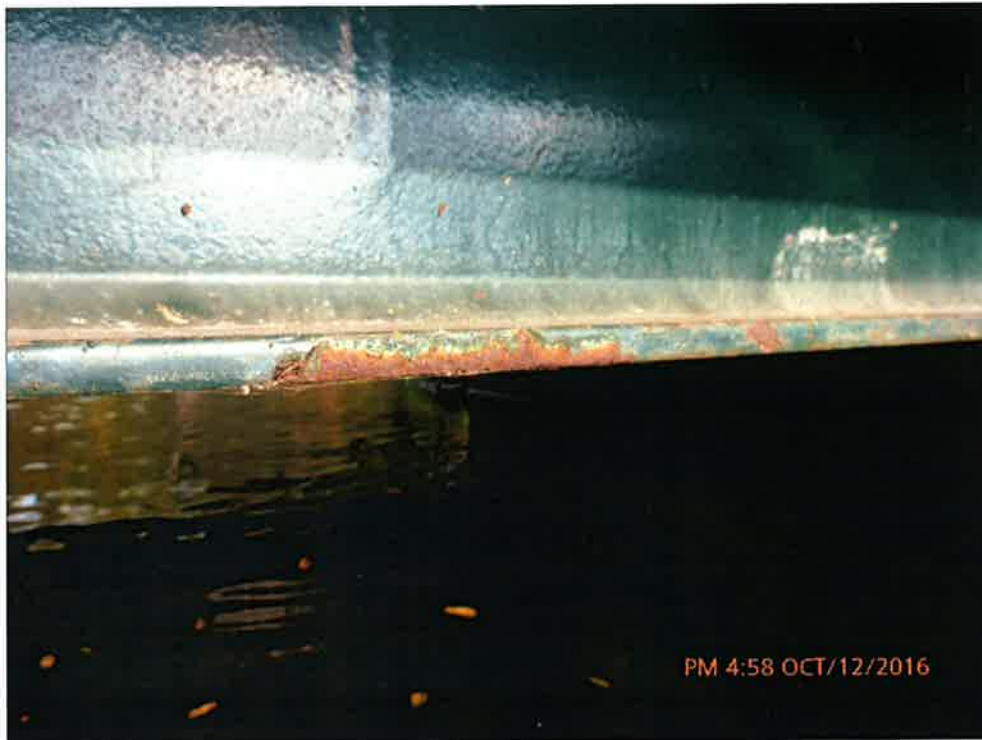
Light Corrosion on Girder
