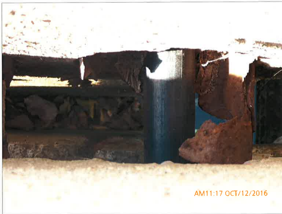
Severely Corroded Utility at Joint
