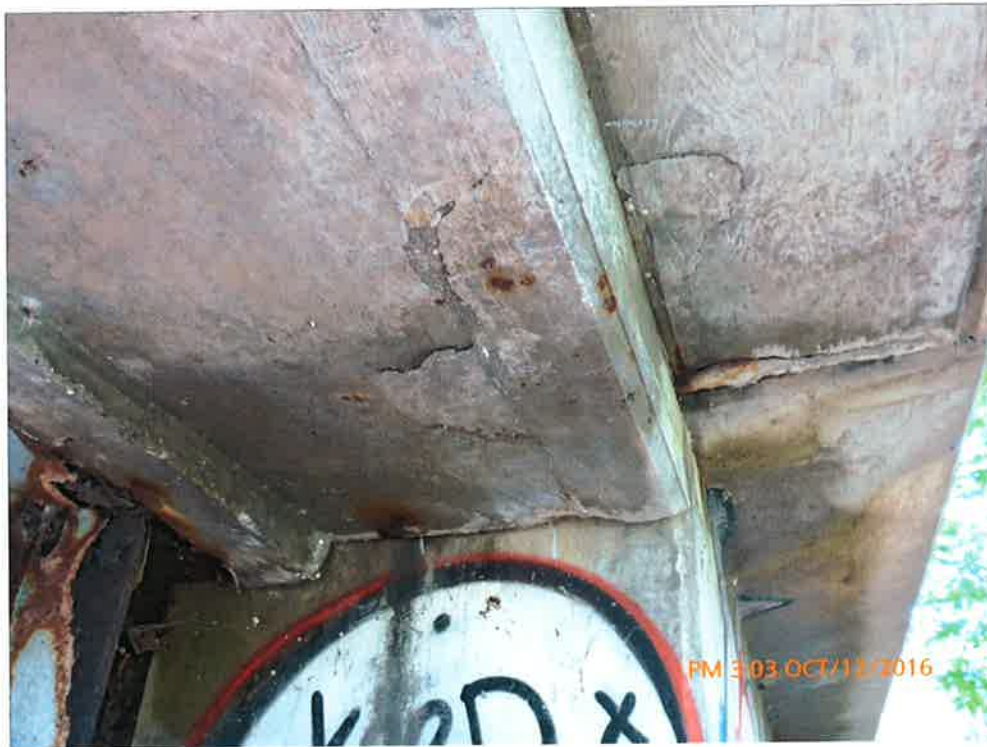
Delamination on End Soffit
