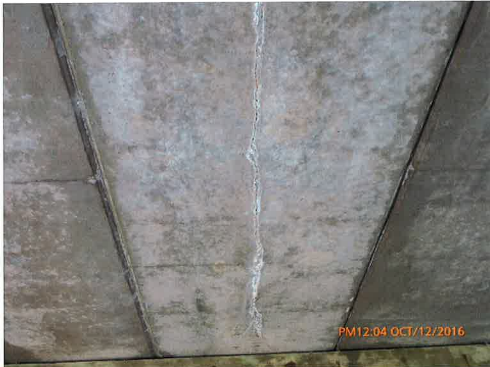
Wide Longitudinal Crack in Box Beam at End
