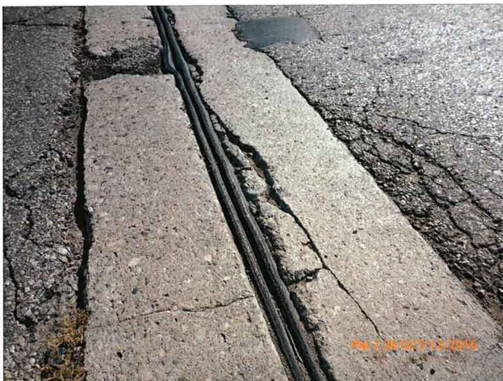
Delamination on Concrete End Dams
