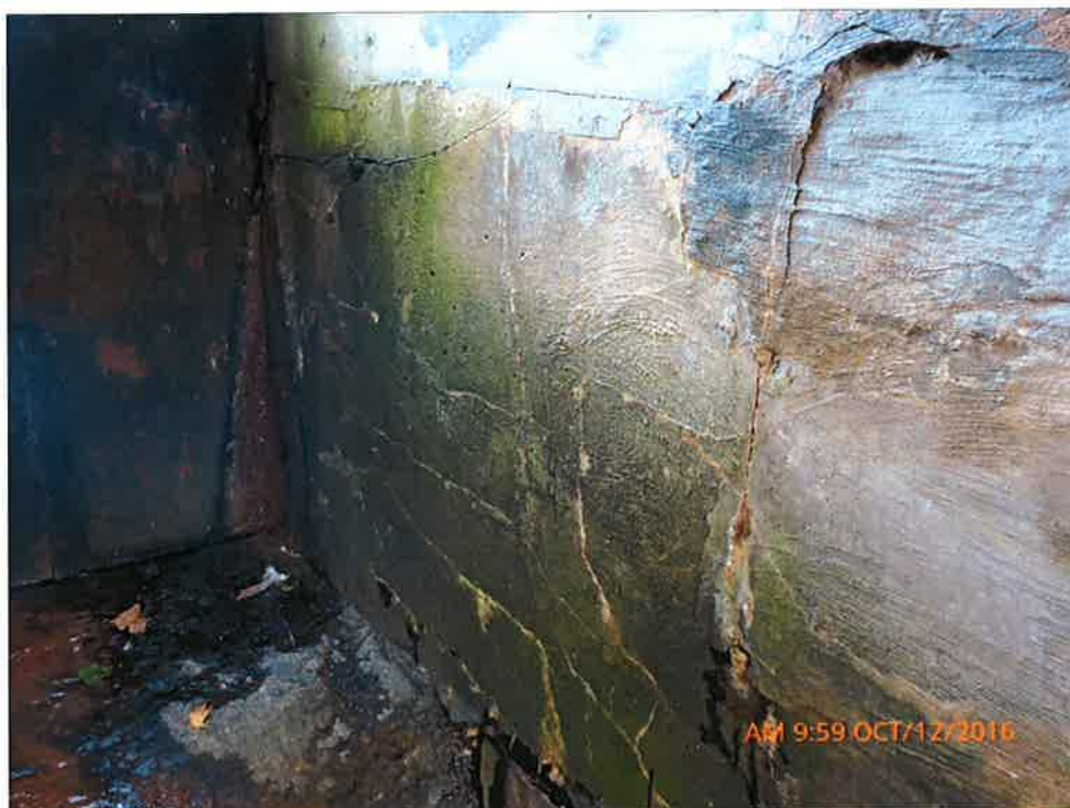
Severe Delamination on Abutment
