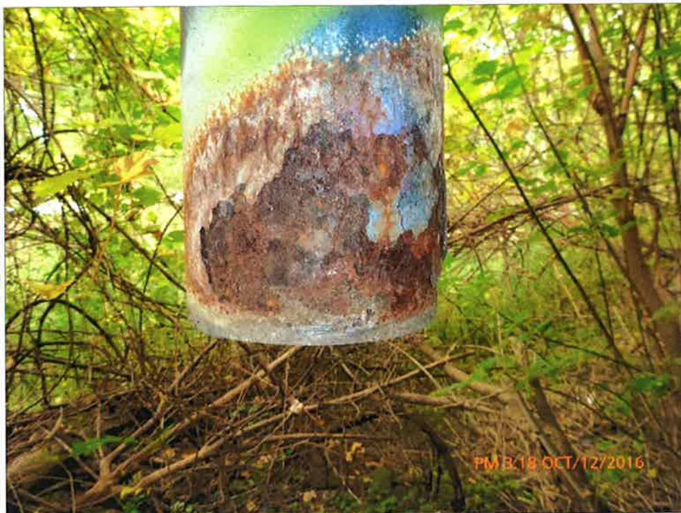
Light Corrosion on Deck Drain
