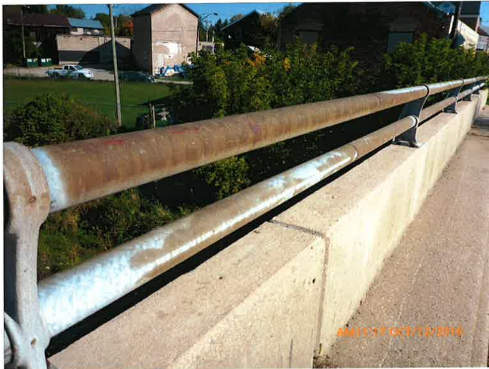
Breakdown of Protective Coating
