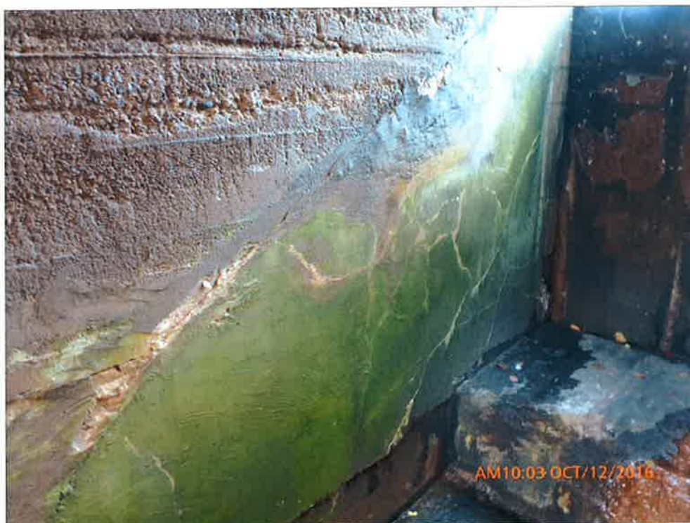
Severe Delamination on Pier
