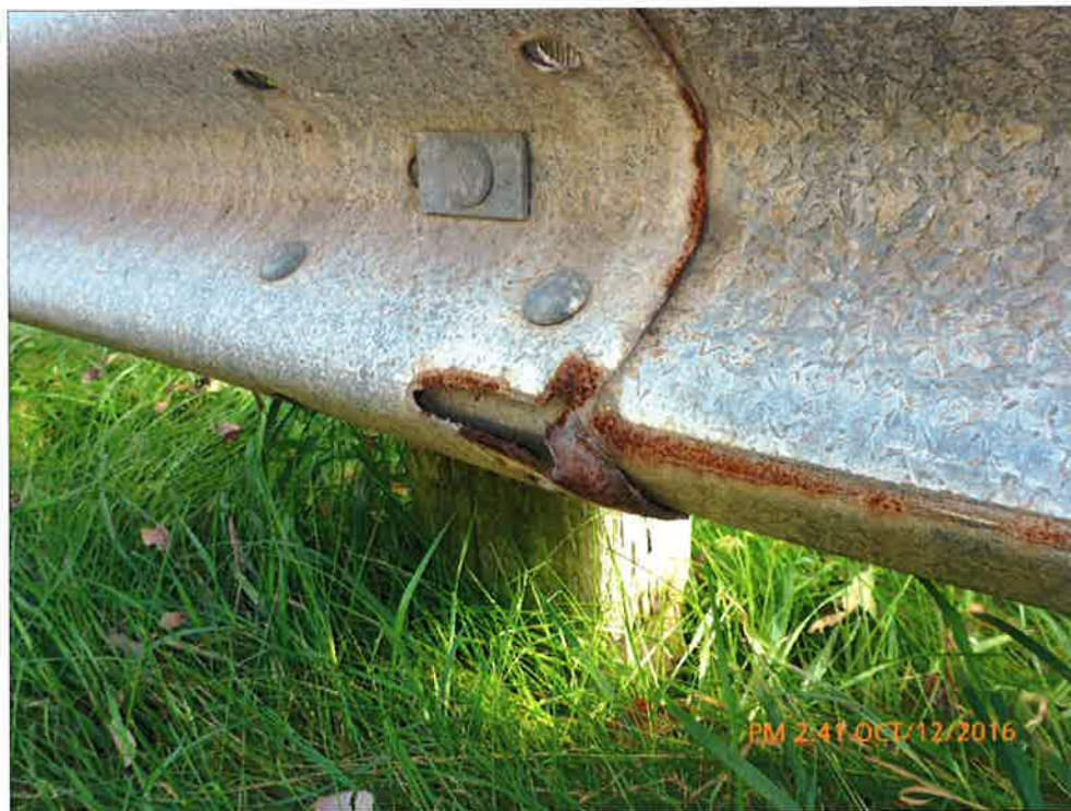
Minor Collision Damage to Guiderail
