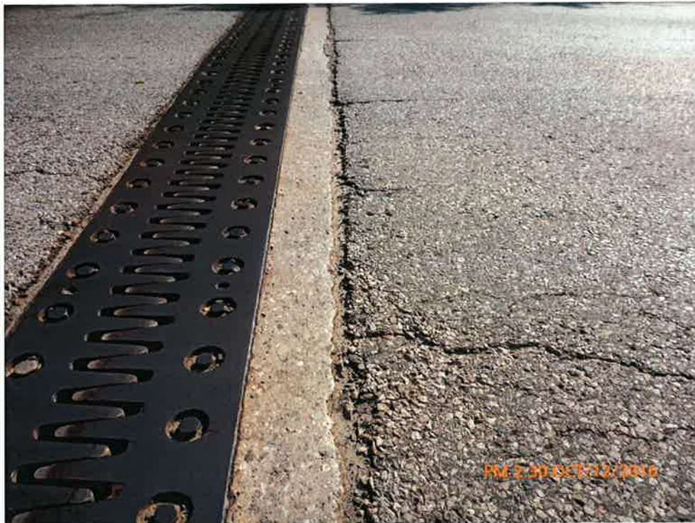
Gap Between End Dam and Approach Wearing Surface
