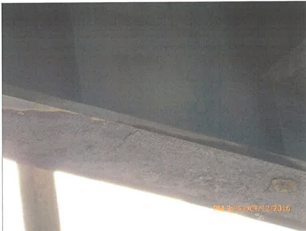
Localized Medium Corrosion on Girder Middle
