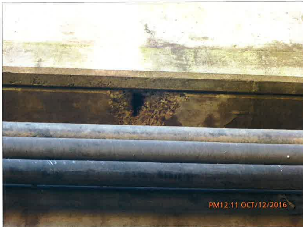
Moderate Spall on Exterior Soffit
