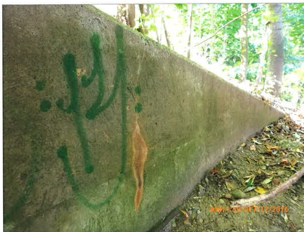
Narrow Stained Crack on Retaining Wall
