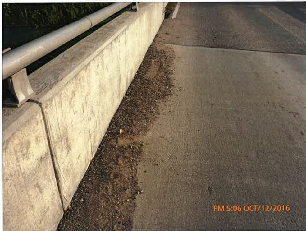
Build-up of Debris on Deck
