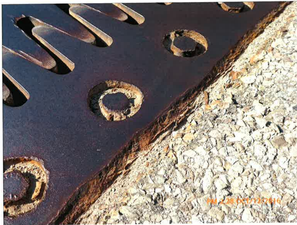
Light Corrosion on Finger Joint
