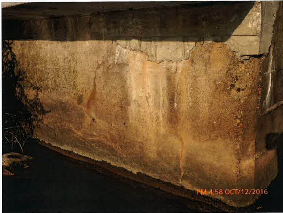
Narrow Stained Crack on Wingwall
