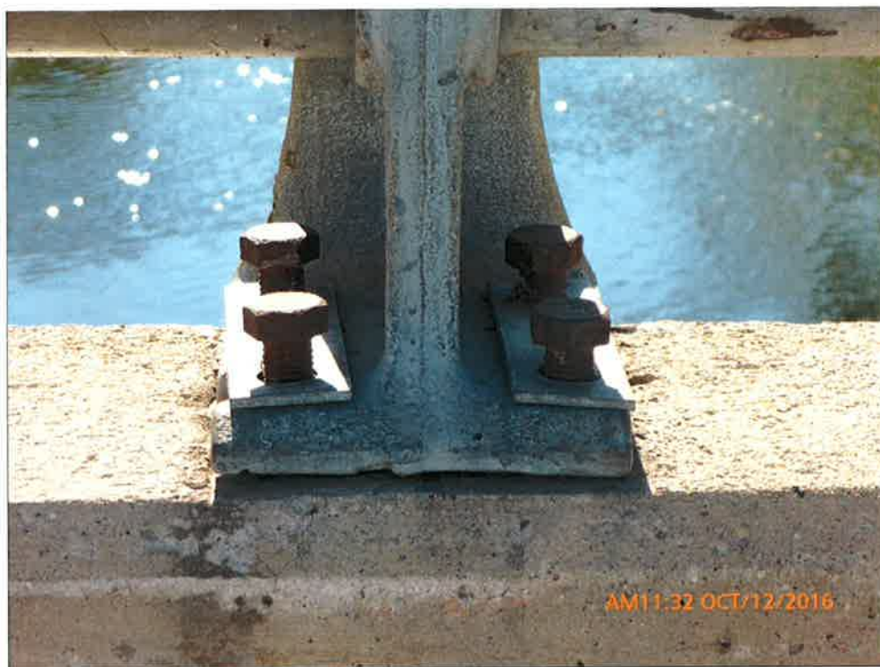
Loose Anchor Bolts on Handrail Post
