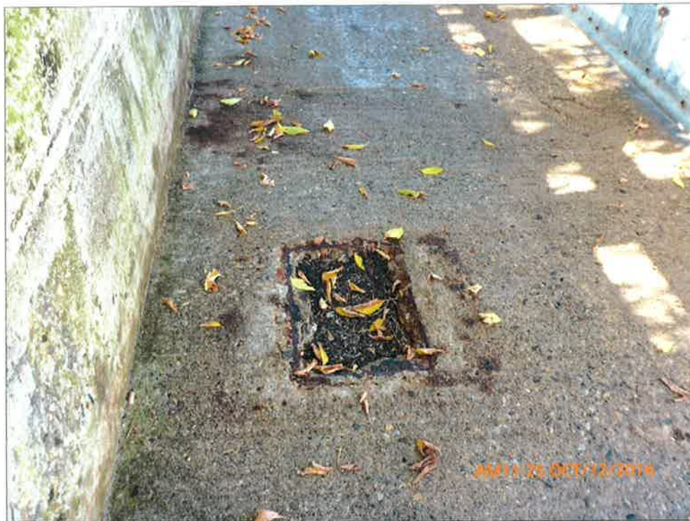
Missing Junction Box Cover Plate in Sidewalk
