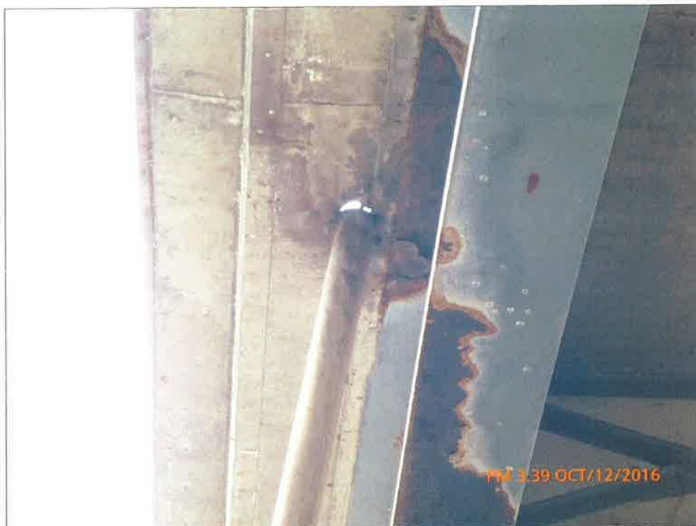
Broken Deck Drain
