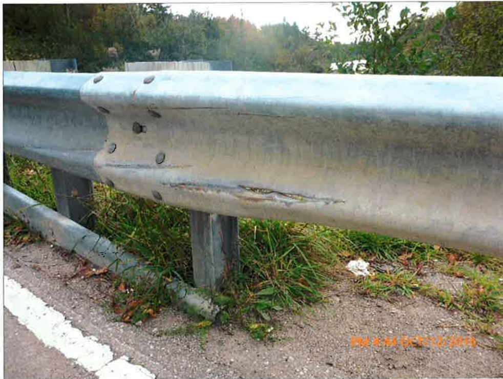
Severe Collision Damage to Guiderail
