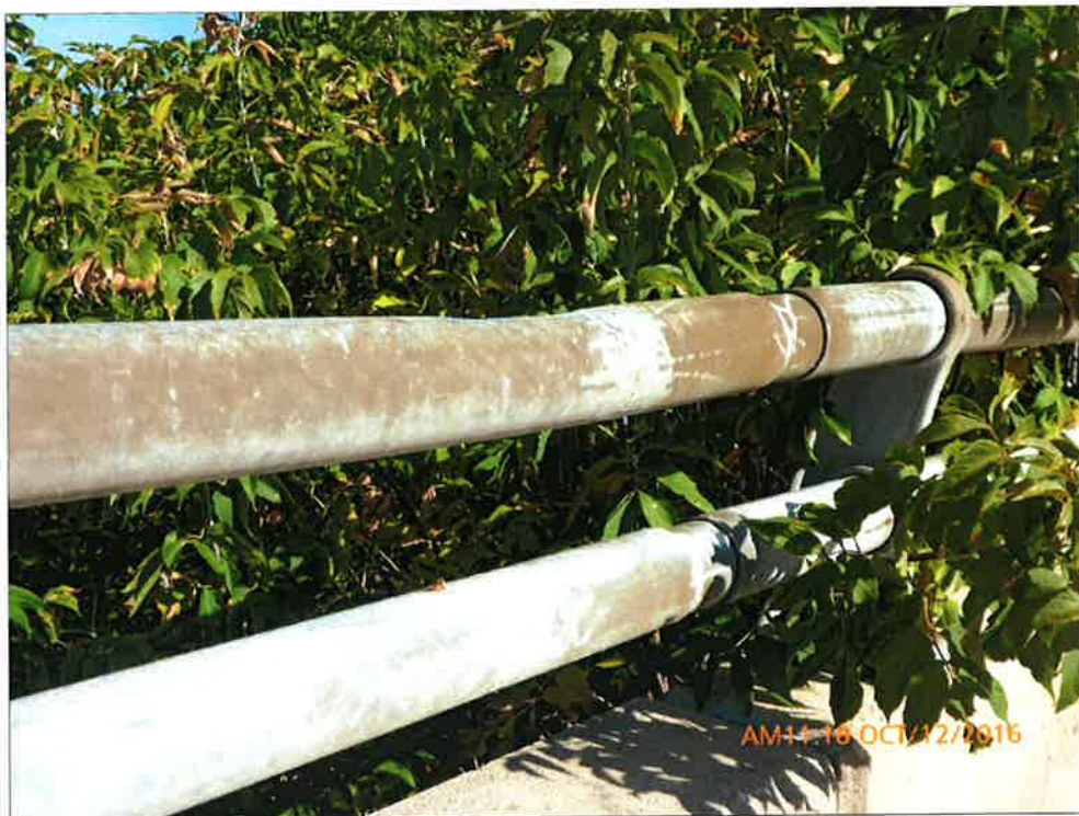
Minor Collision Damage to Handrail
