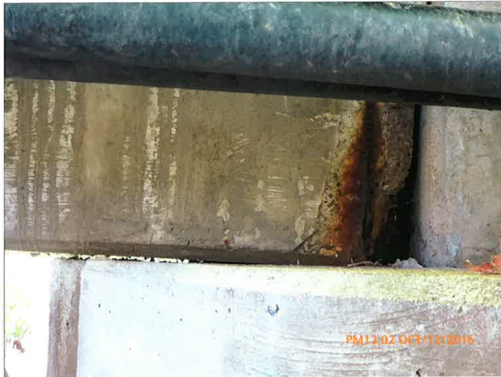
Squashed Abutment Bearing
