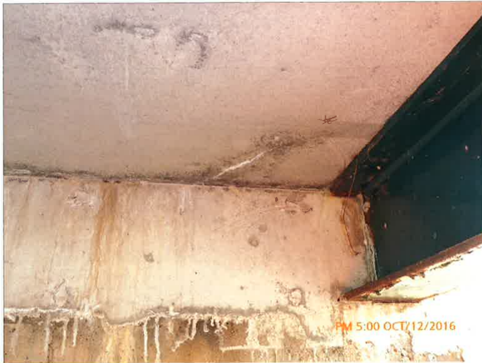
Narrow Stained Crack on Interior Soffit
