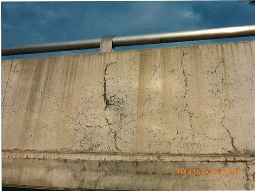
Narrow Stained Cracks on Exterior Parapet Wall
