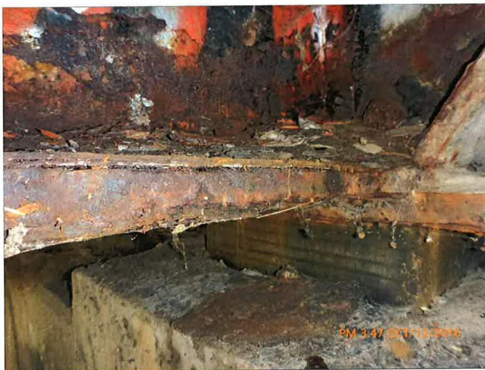
Severe Corrosion on End Girder
