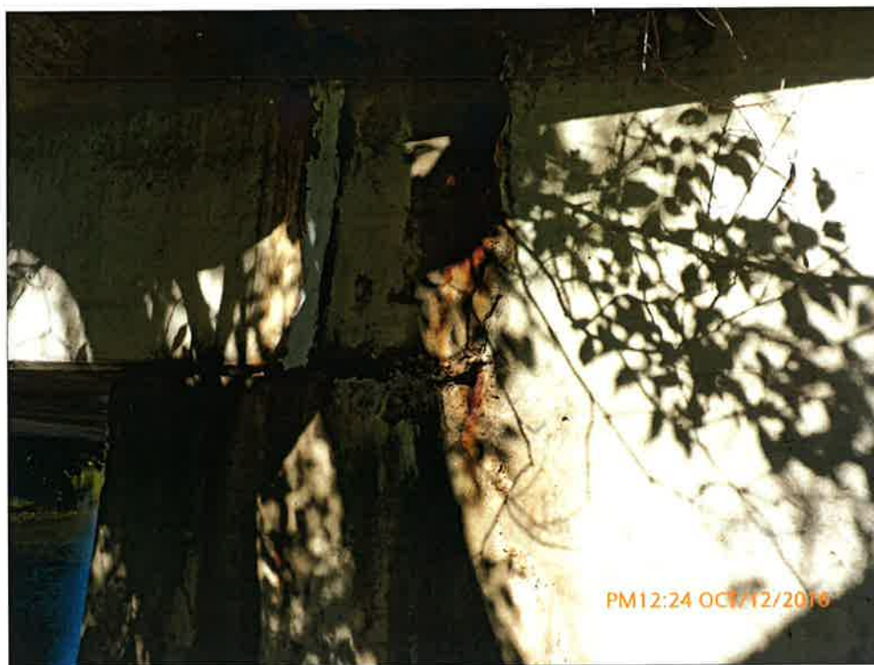
Narrow Stained Crack on Southeast Wingwall
