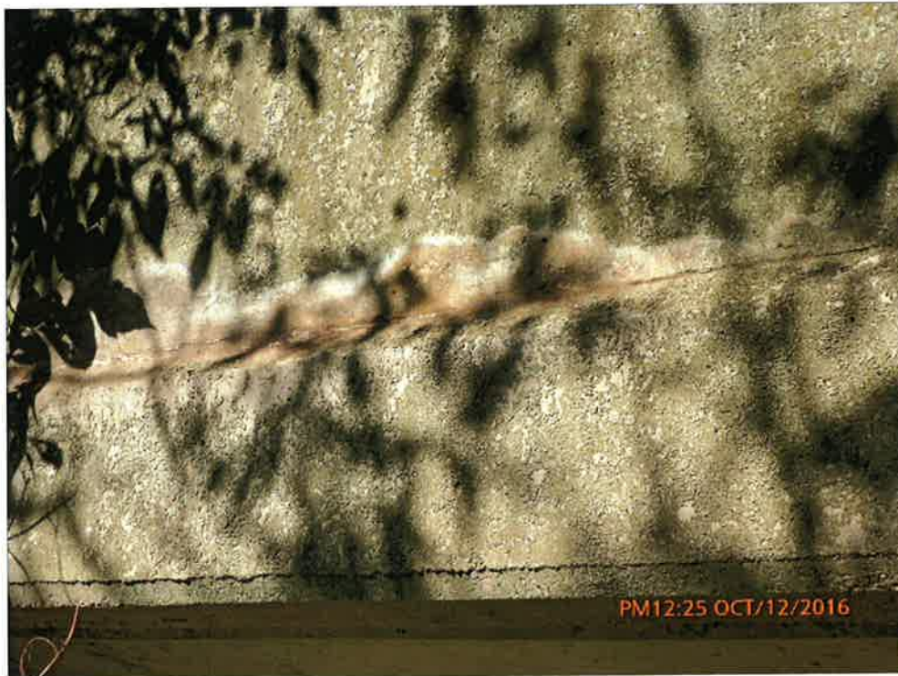
Narrow Stained Crack on Exterior Parapet Wall
