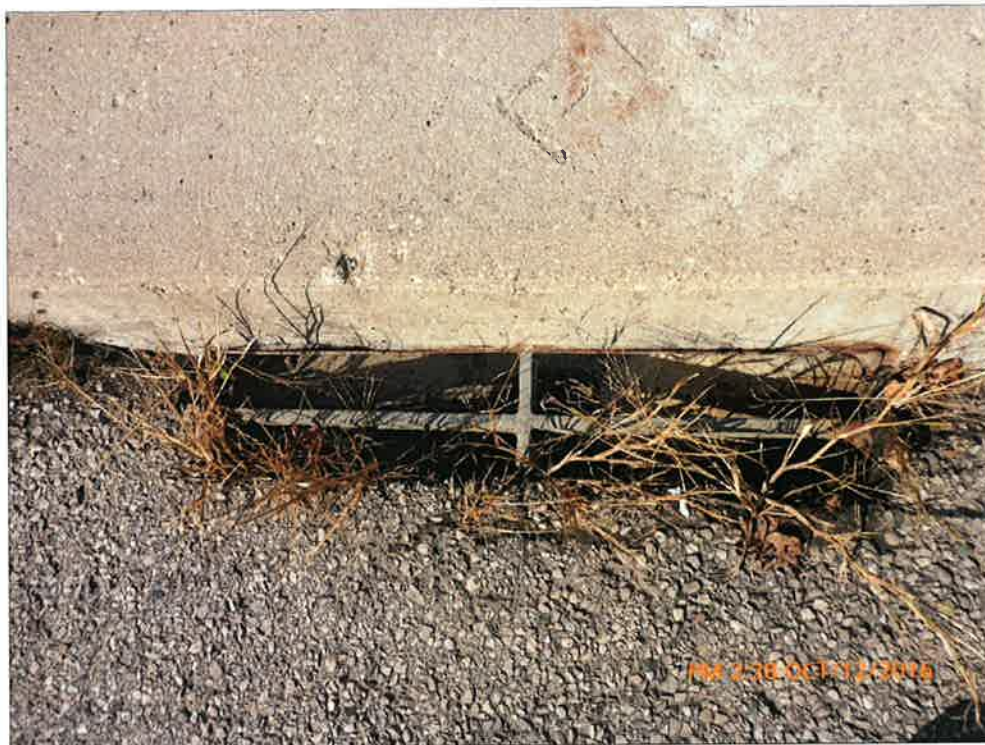
Broken Deck Drain
