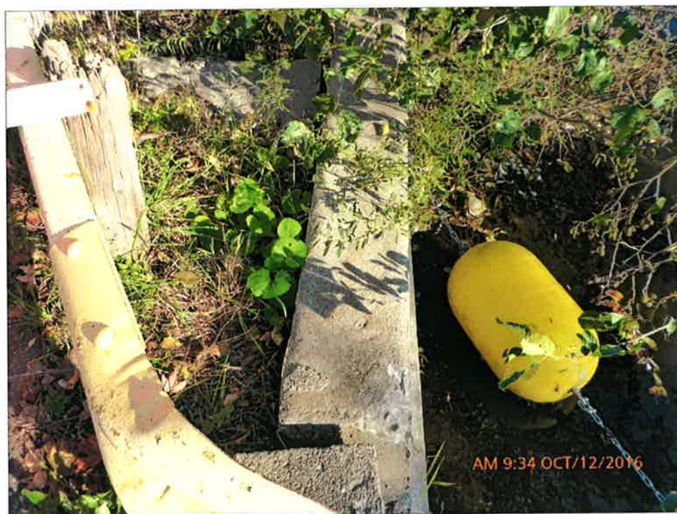
Minor Outward Rotation of Retaining Wall
