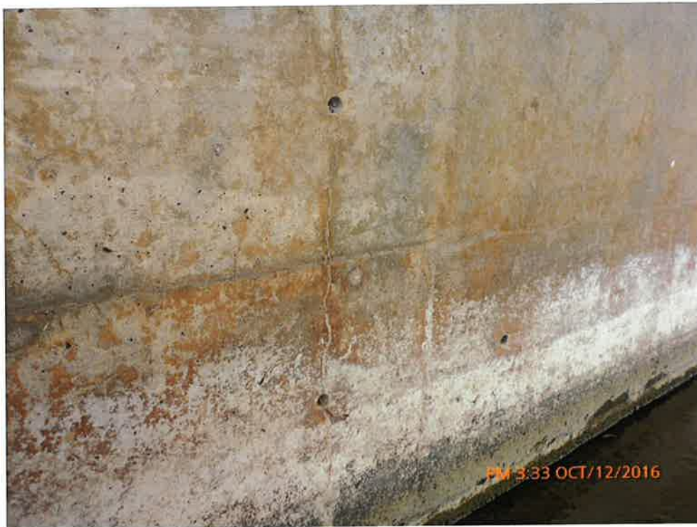
Narrow Stained Crack on Pier
