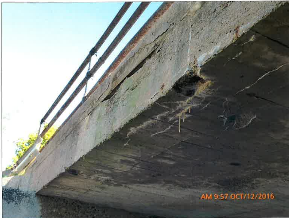
Light Spall on Exterior Soffit
