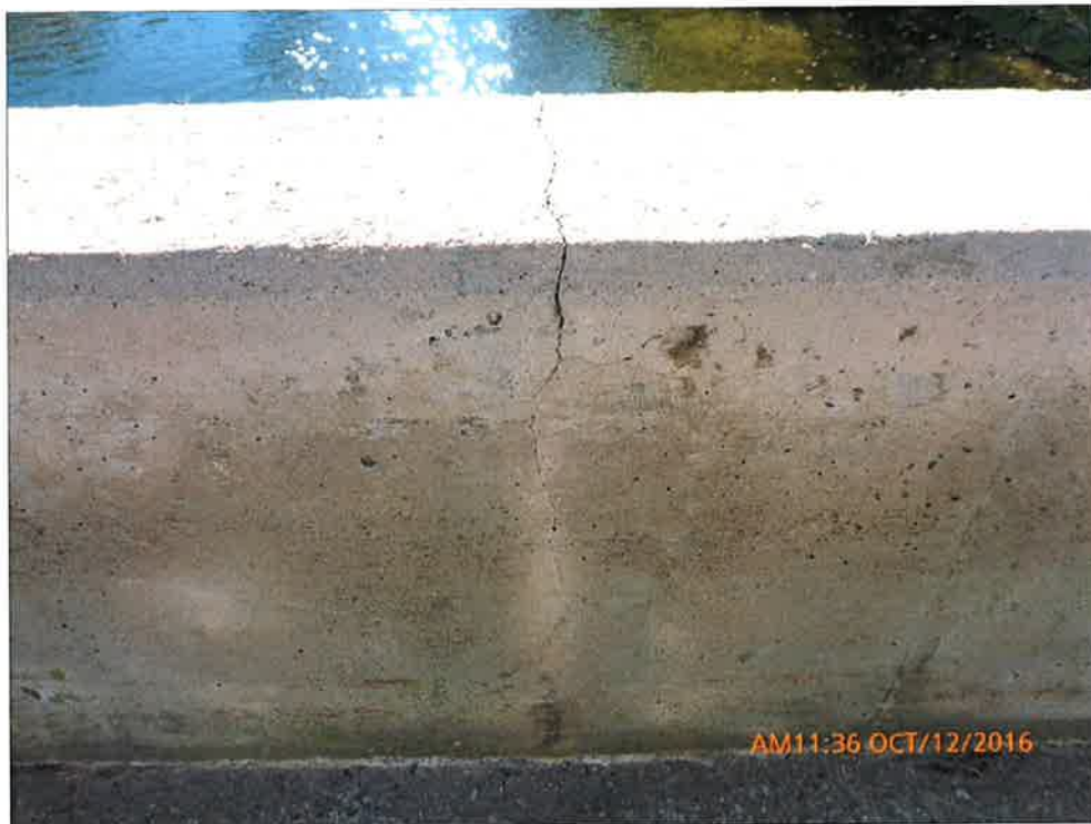
Narrow Stained Crack on Interior Parapet Wall
