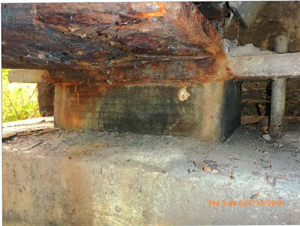
Typical West Abutment Bearing
