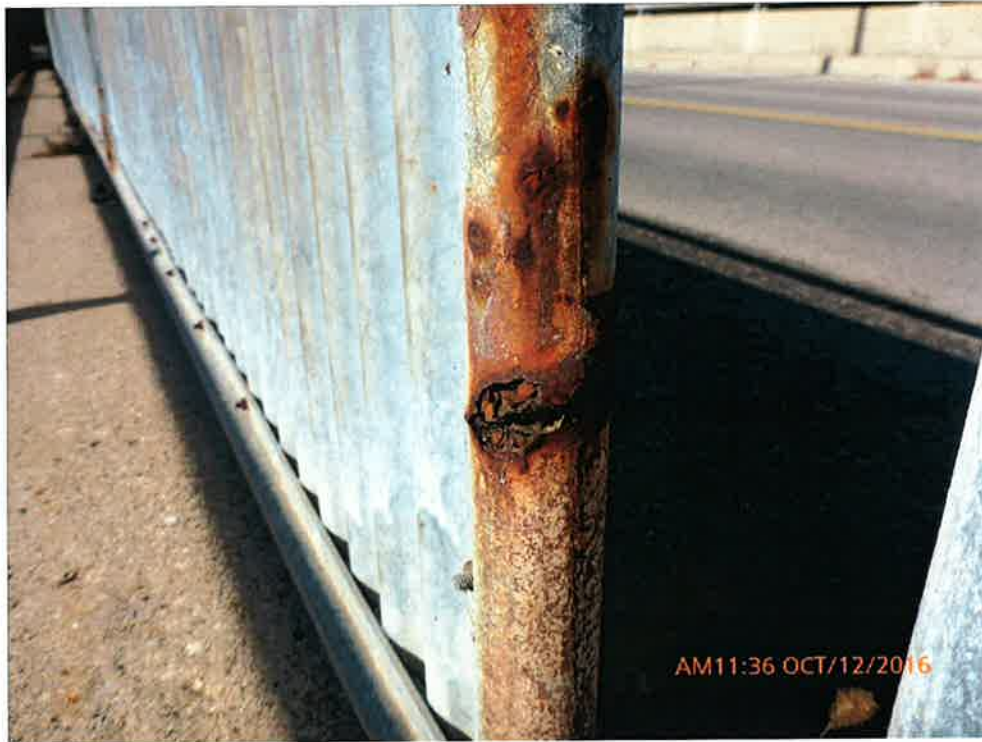
Perforation on Pedestrian Splash Barrier
