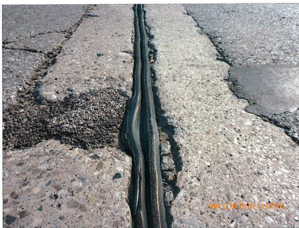
Displaced Seal
