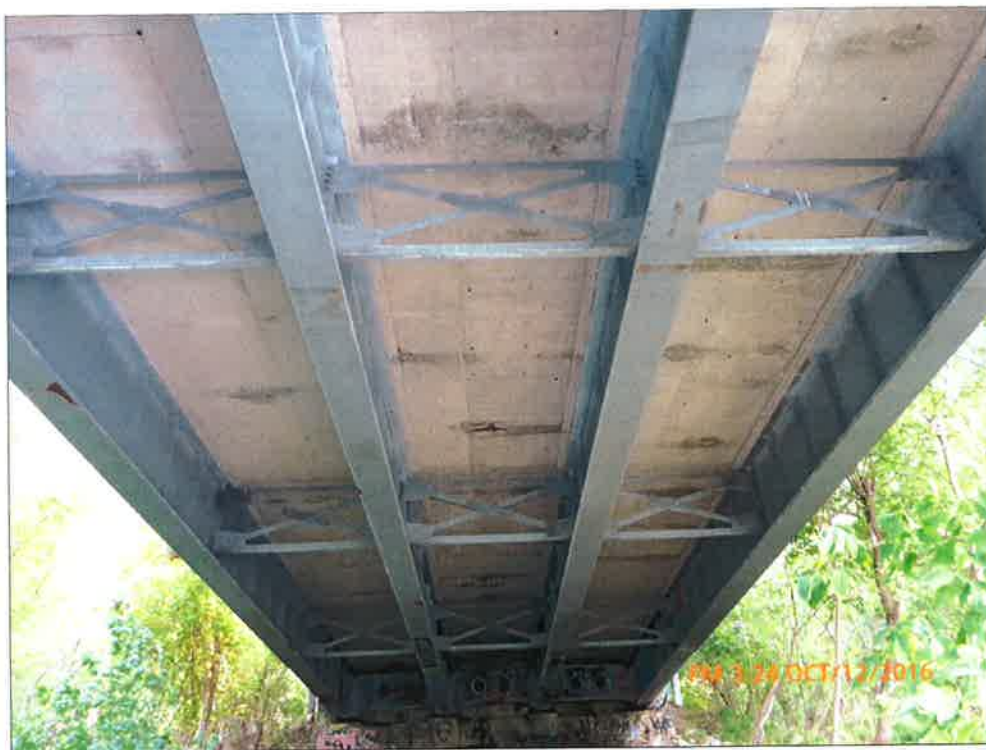
Typical End Span Soffit
