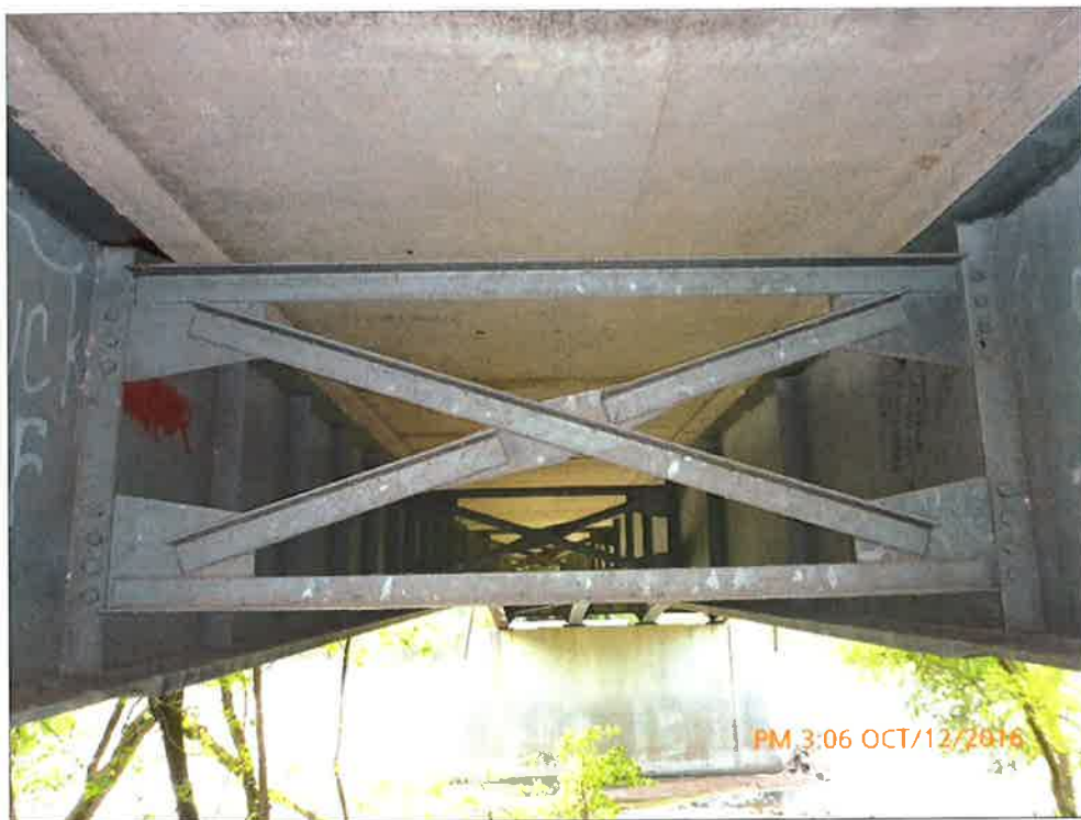
Typical Intermediate Diaphragm
