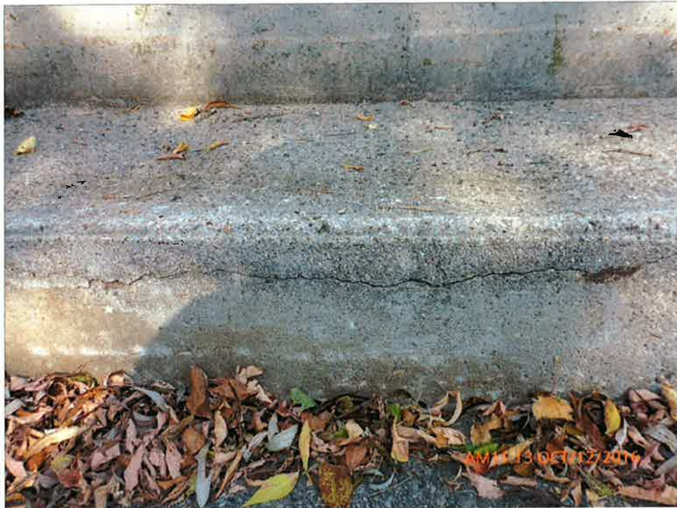
Delamination on Curb
