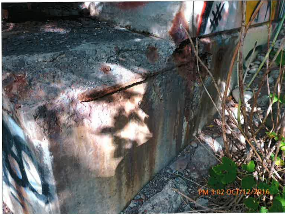
Spall on Wingwall
