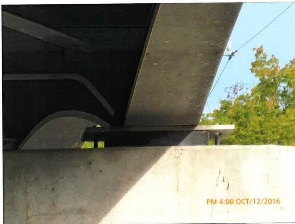
Typical Pier Bearing
