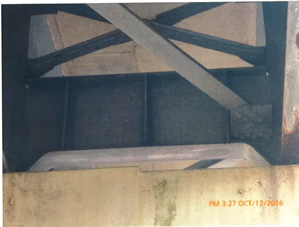
Typical Diaphragm at Pier
