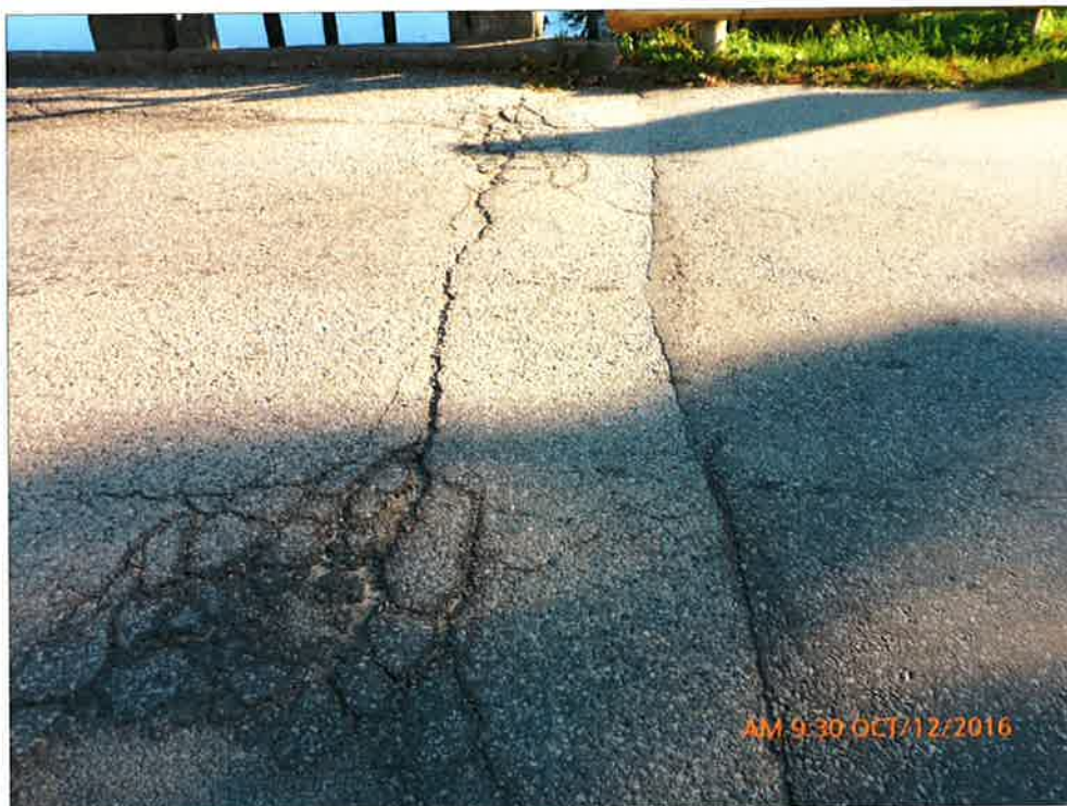
Wide Crack in Approach Wearing Surface
