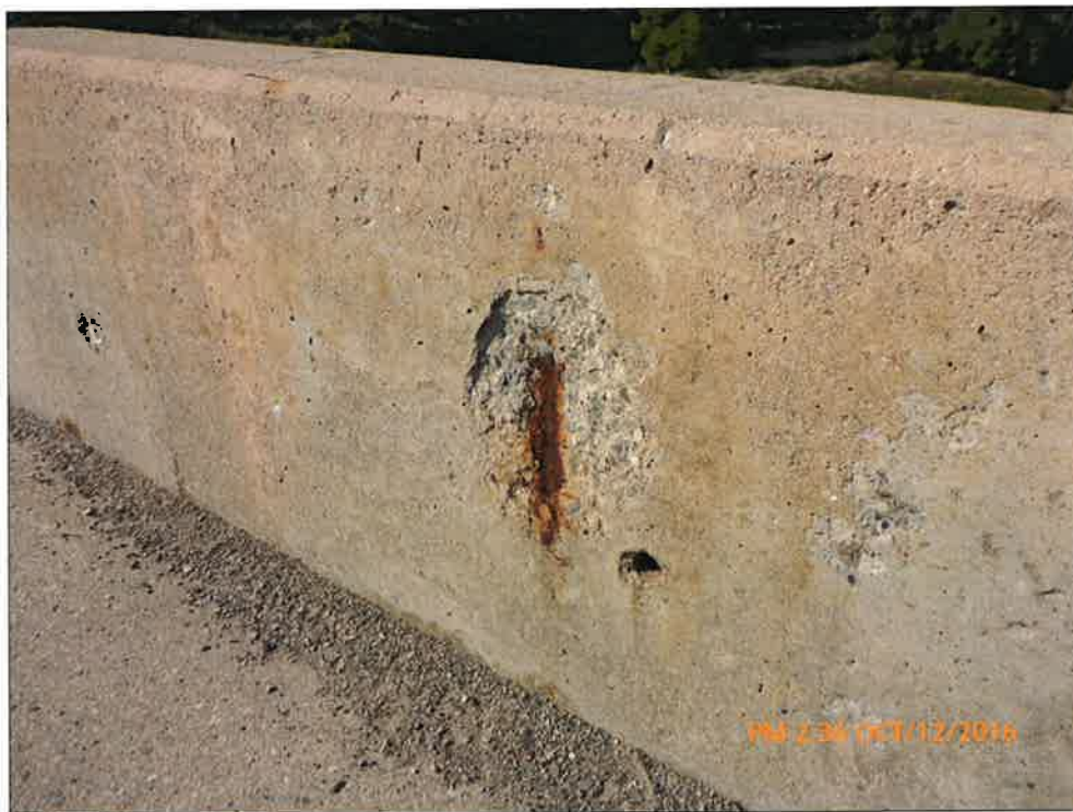
Light Spall on Interior Parapet Wall
