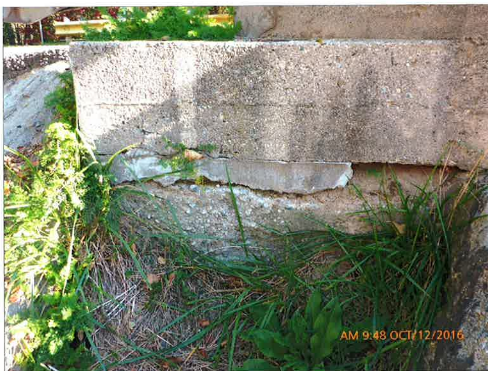
Debonded Concrete Patch on Wingwall
