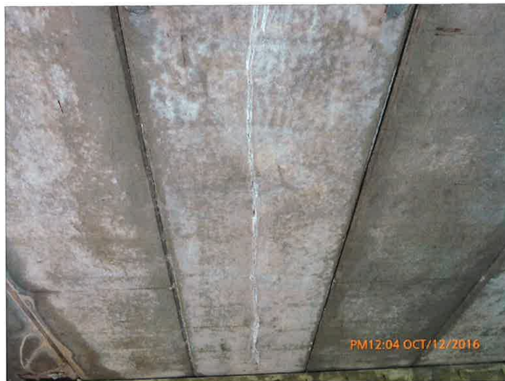
Wide Longitudinal Crack in Box Beam Middle
