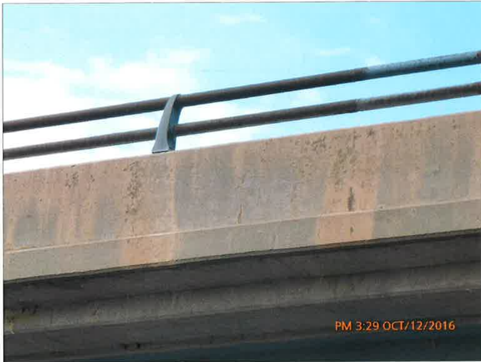
Narrow Stained Cracks on Exterior Parapet Wall
