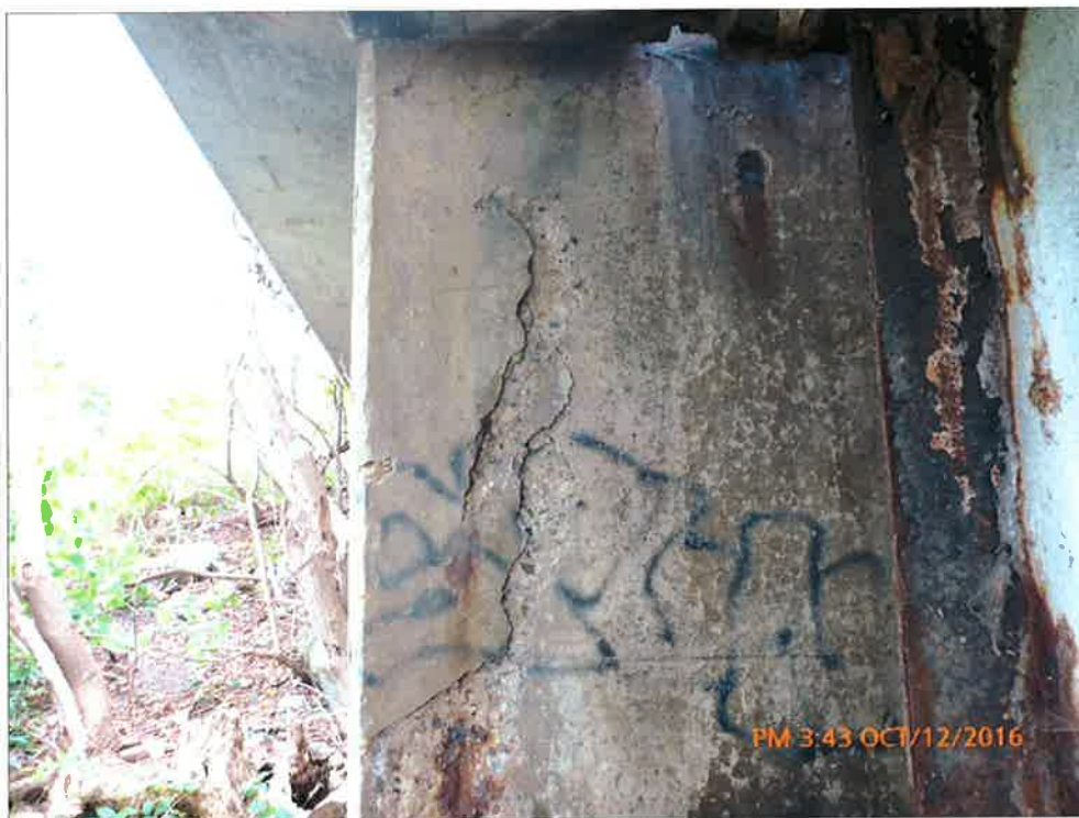
Delamination on Ballast Wall
