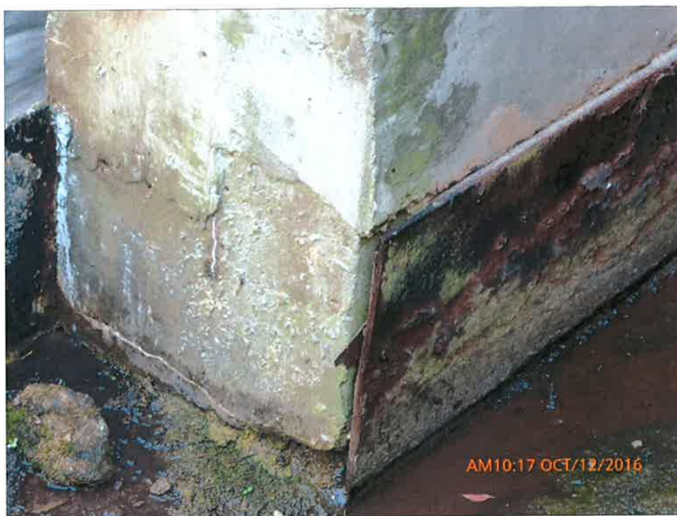
Light Corrosion on Splash Guard
