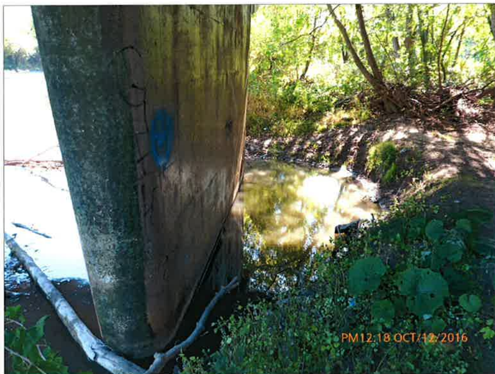
Minor Erosion Around West Pier
