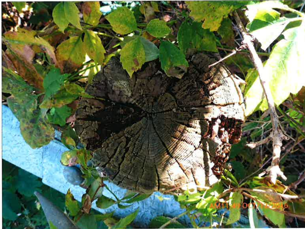
Moderate Weathering of Guiderail Post
