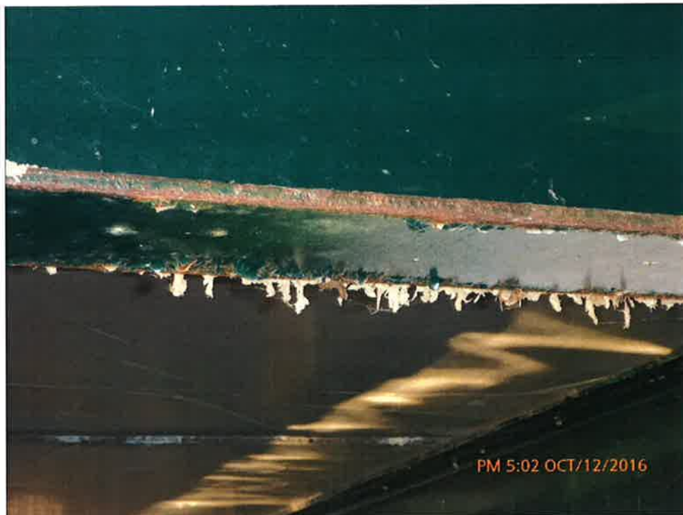
Breakdown of Protective Coating
