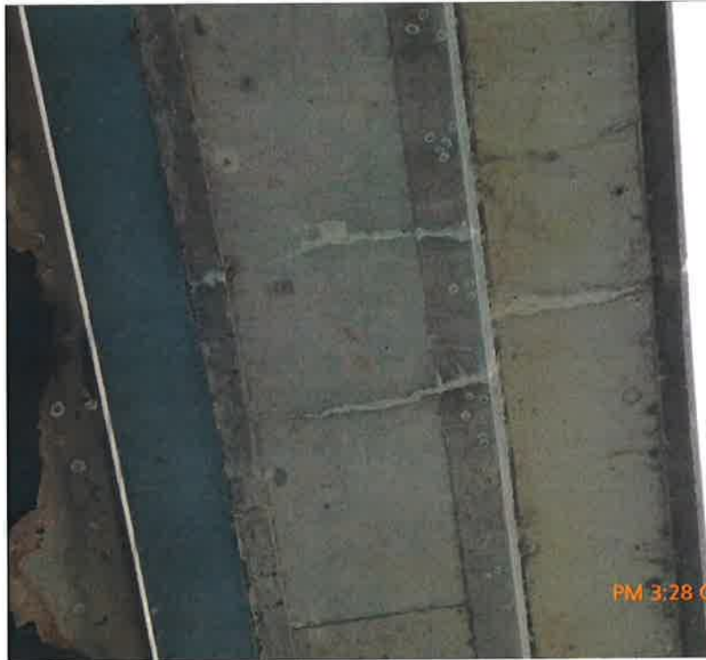
Narrow Stained Cracks on Exterior Soffit
