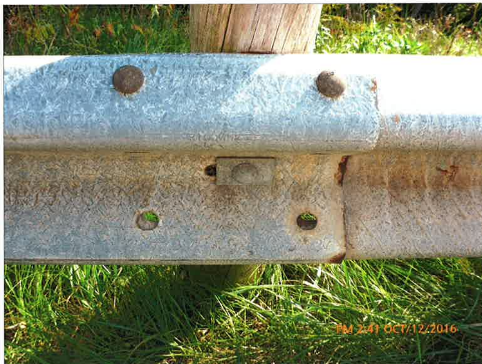
Missing Bolts on Guiderail
