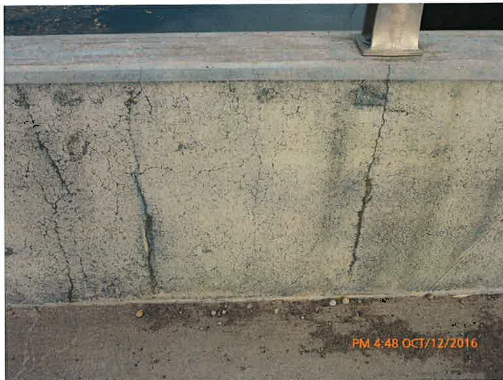
Narrow Stained Cracks on Interior Parapet Wall
