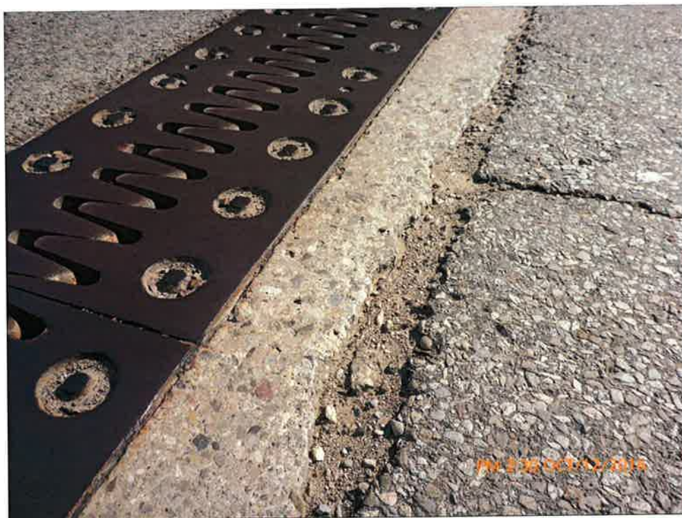
Moderate Abrasions on Concrete End Dam
