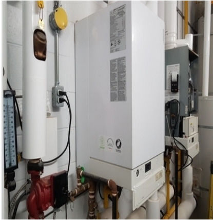
(a) Condensing boiler
