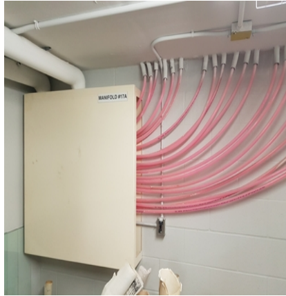
(b) Infloor radiant heating manifold
