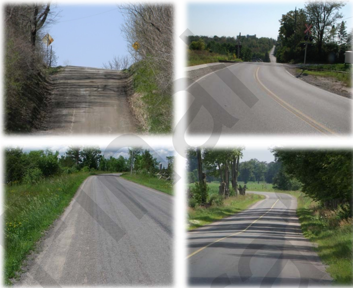
Figure 3.2: Potentially Substandard Vertical and Horizontal Alignment
