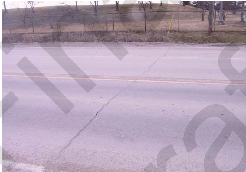
Transverse /Thermal cracking
