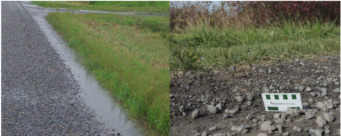
Figure 3.4: Poor Shoulder Drainage
