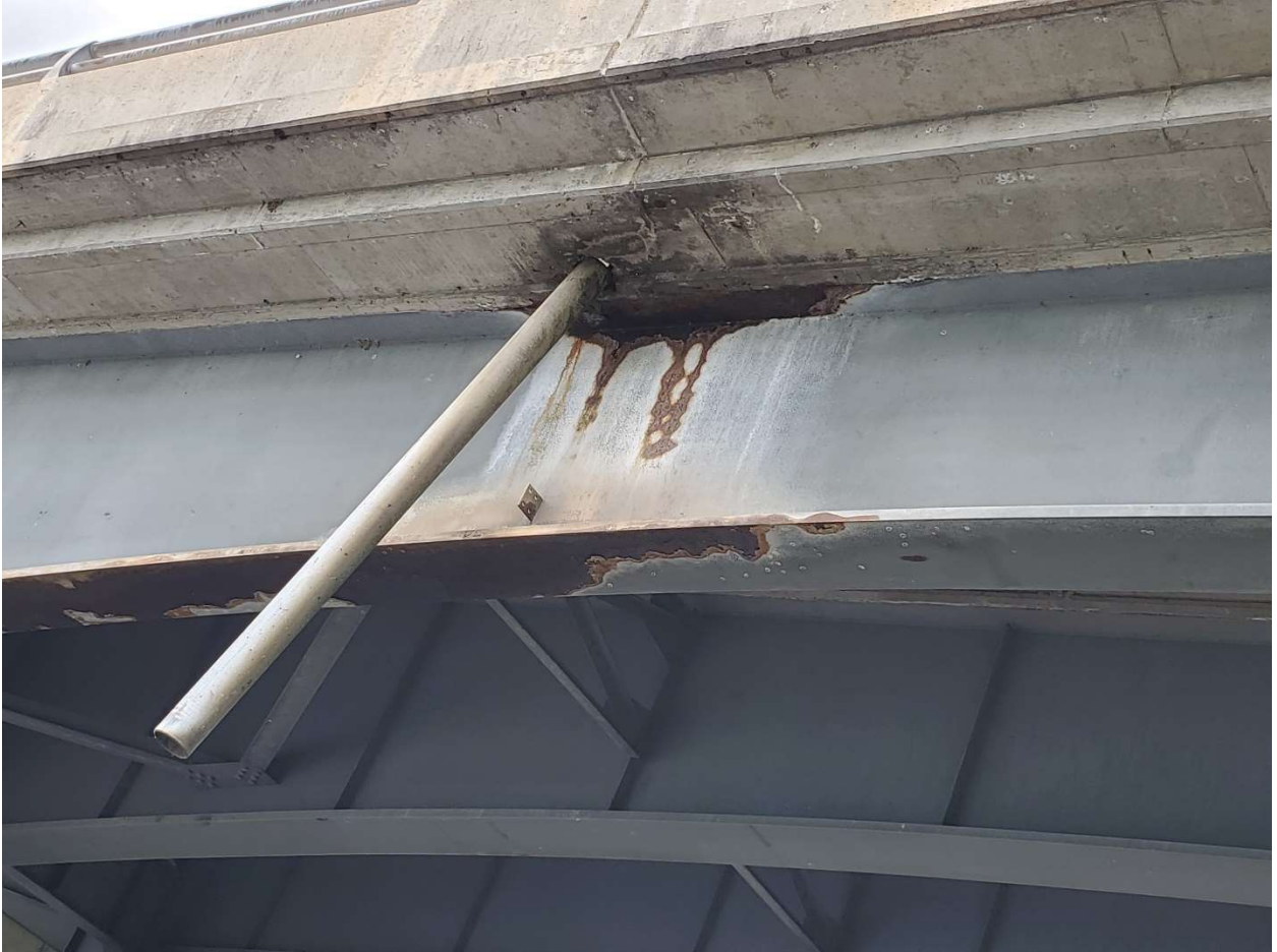
Damaged drain pipe and corrosion in the surrounding area
