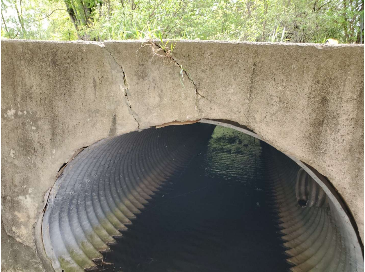
Multiple cracks observed in the concrete
