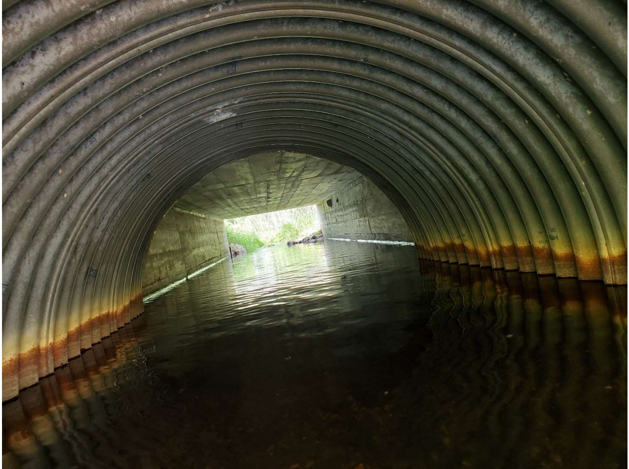
Rusting observed at the culvert bottom
