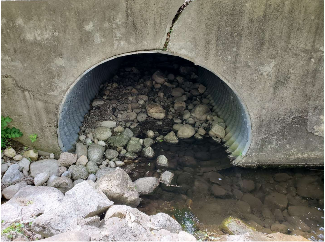
Large crack observed on the concrete
