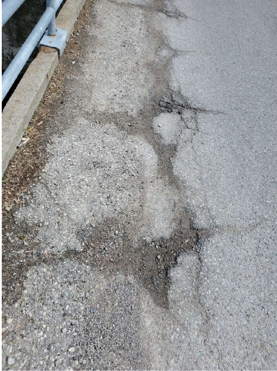
Damage observed on the wearing surface of the bridge
