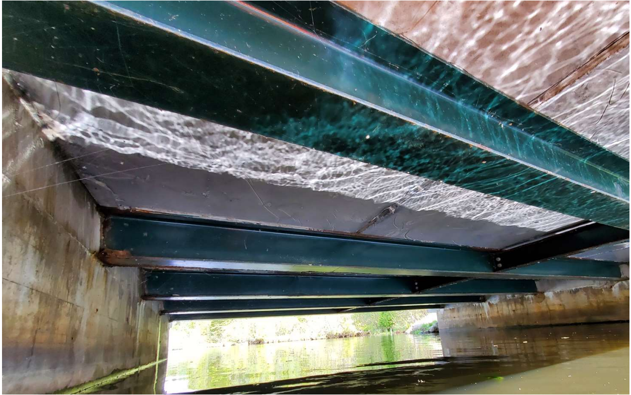
Steel girders underneath the bridge
