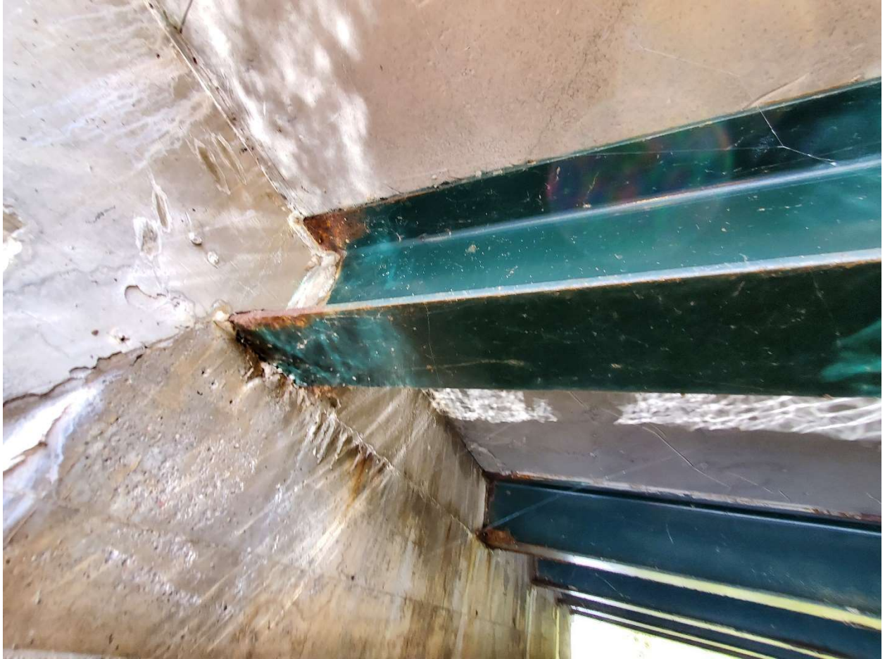
Rusting observed at the girder ends
