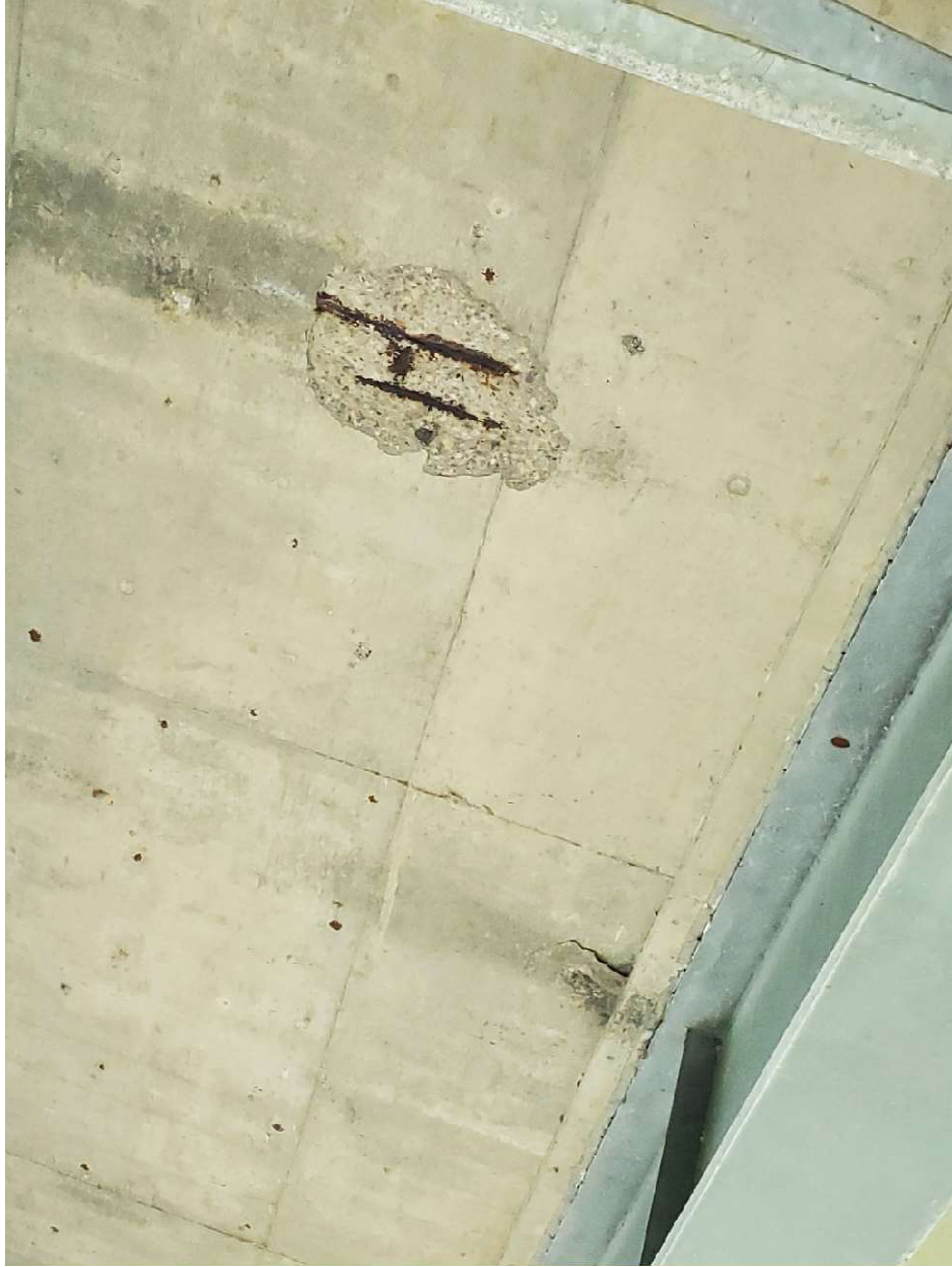
Spalling of concrete/ Exposed Rebar observed in Soffit
