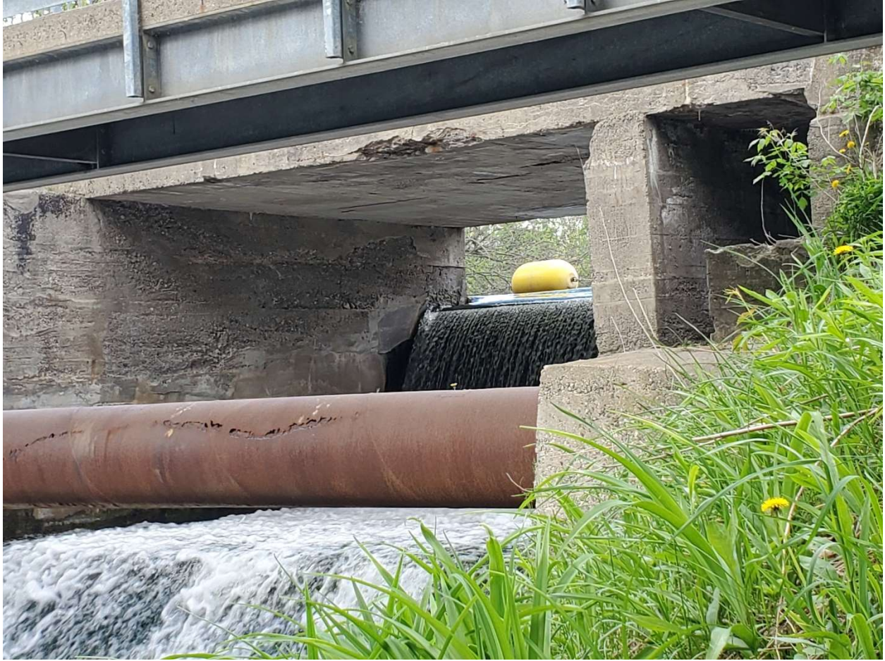
Crack and spalling observed in the concrete slab
