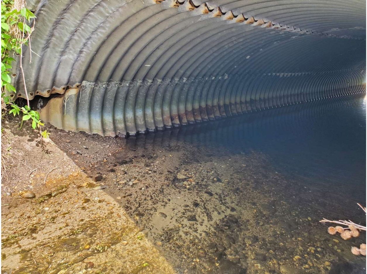
Rusting observed at Culvert joints
