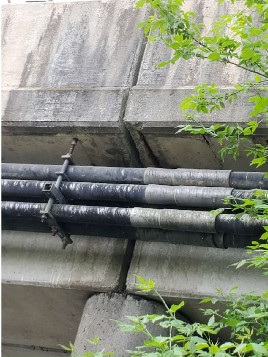
Damages observed at the Abutment
