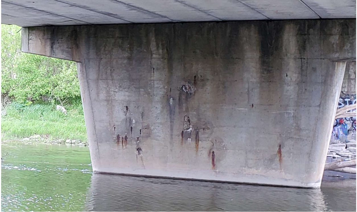
Exposed reinforcement and spalling at the West pier
