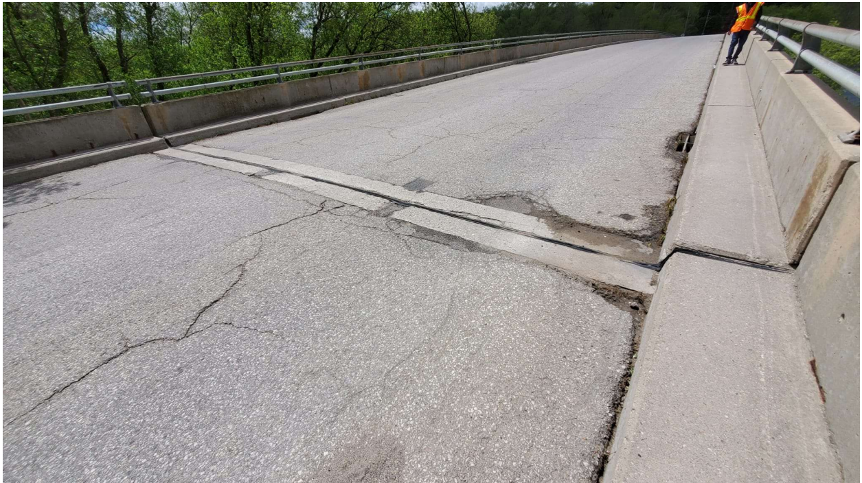
Expansion joints at the East Approach
