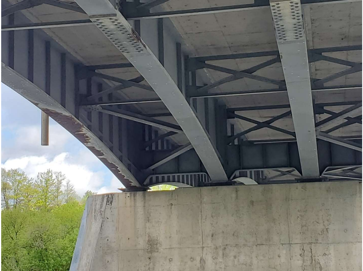
Rusting observed in one of the bridge girders
