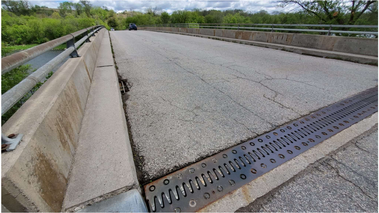
Expansion joints at the West Approach
