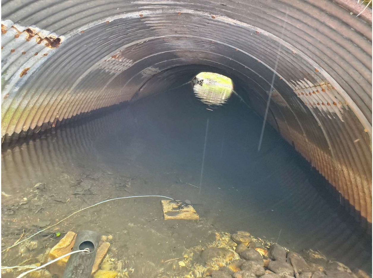
Some rusting observed in the culvert
