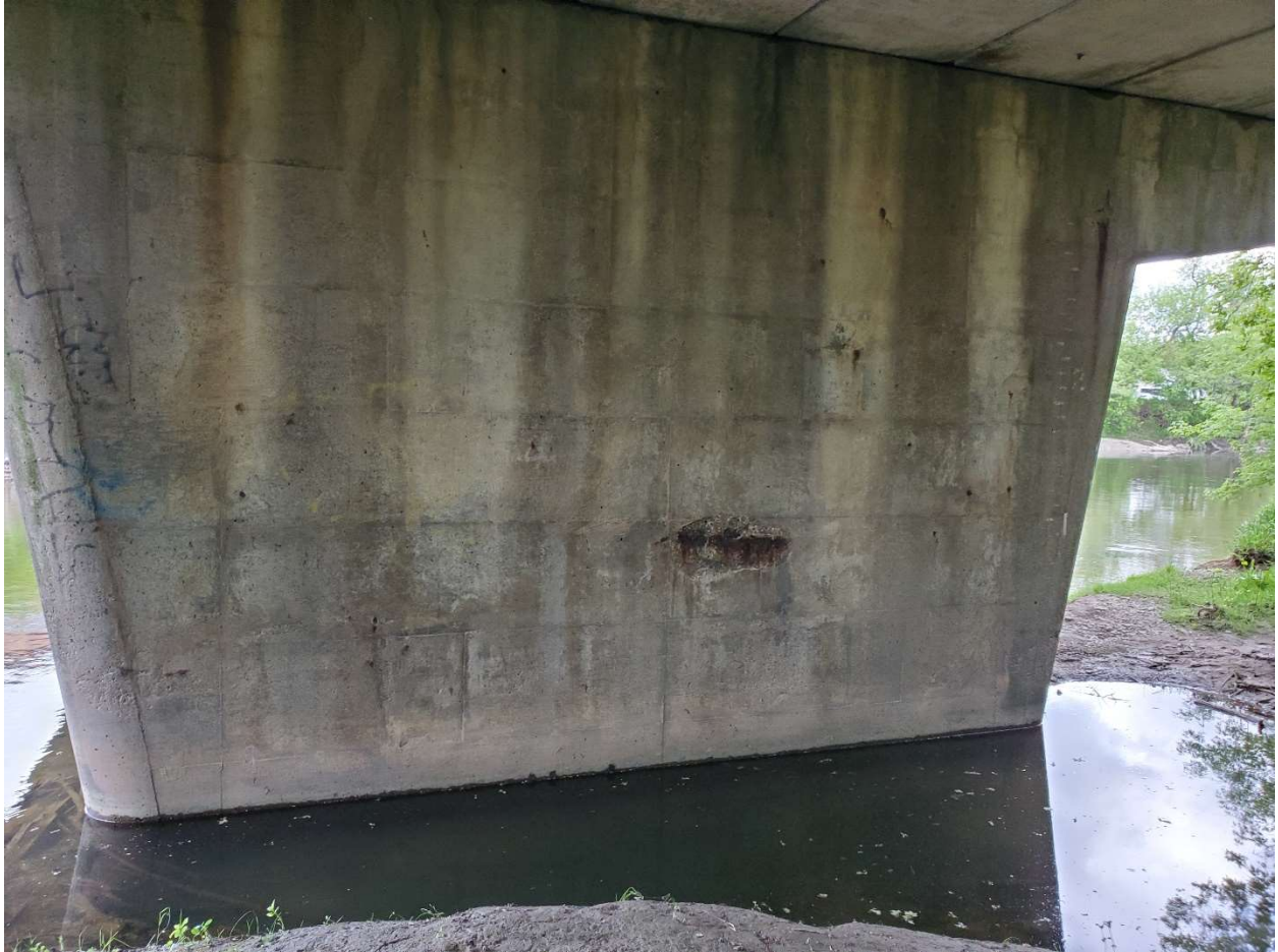
Exposed reinforcement and spalling at the East pier
