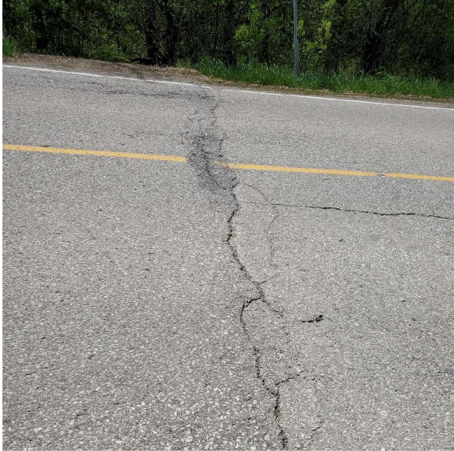
Some cracks observed in the wearing surface of the road
