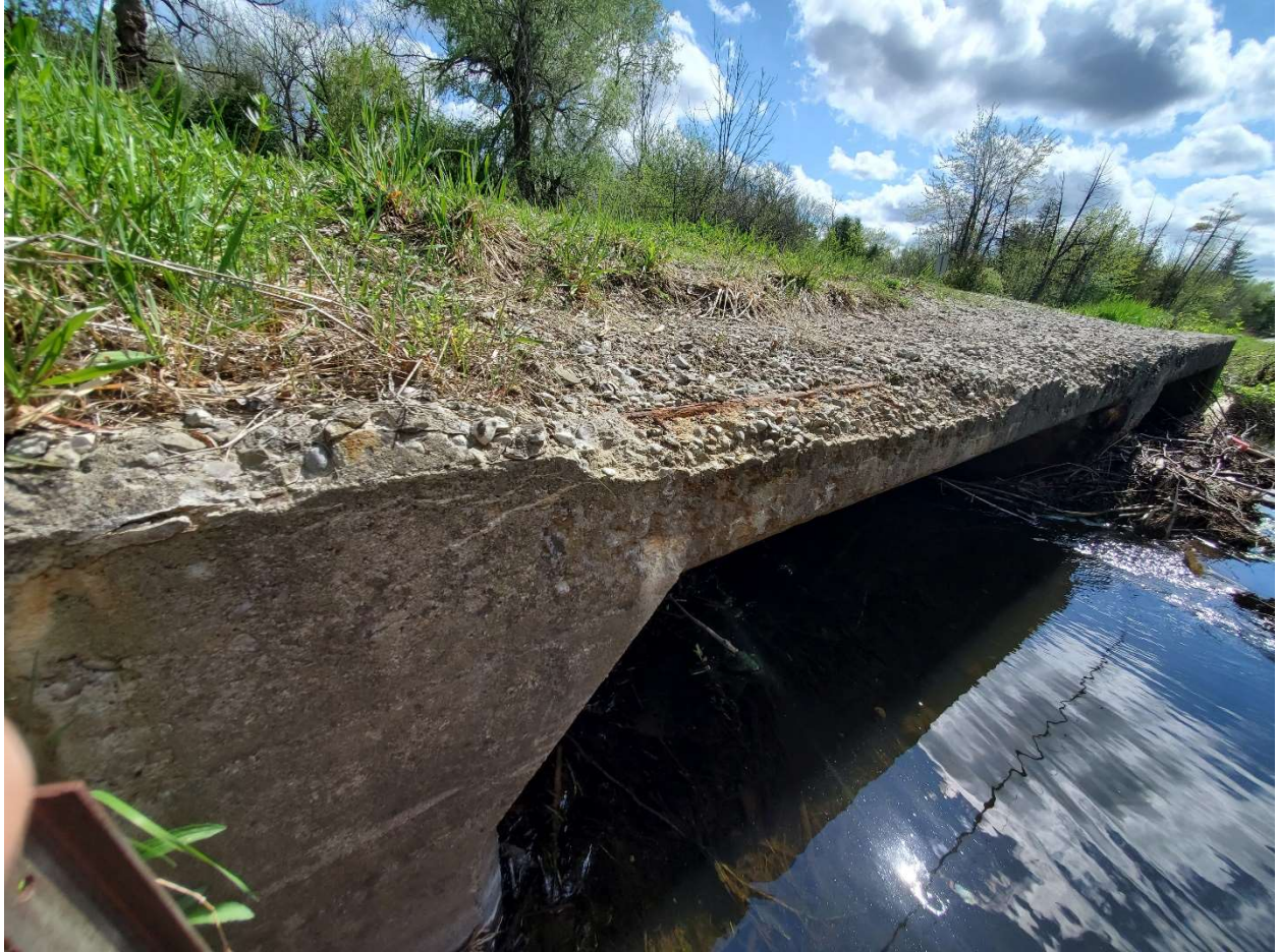
Exposed rebar on the top of the box culvert
