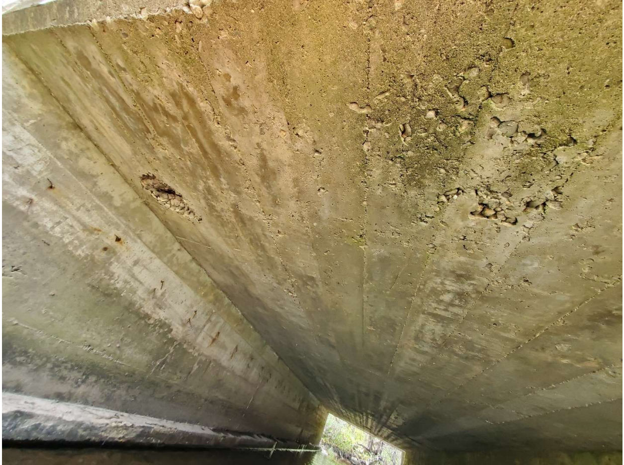
Concrete honeycomb and spalling observed inside the culvert
