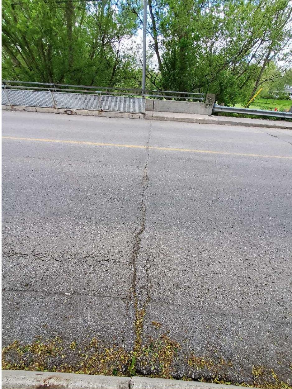
Deterioration the deck surface
