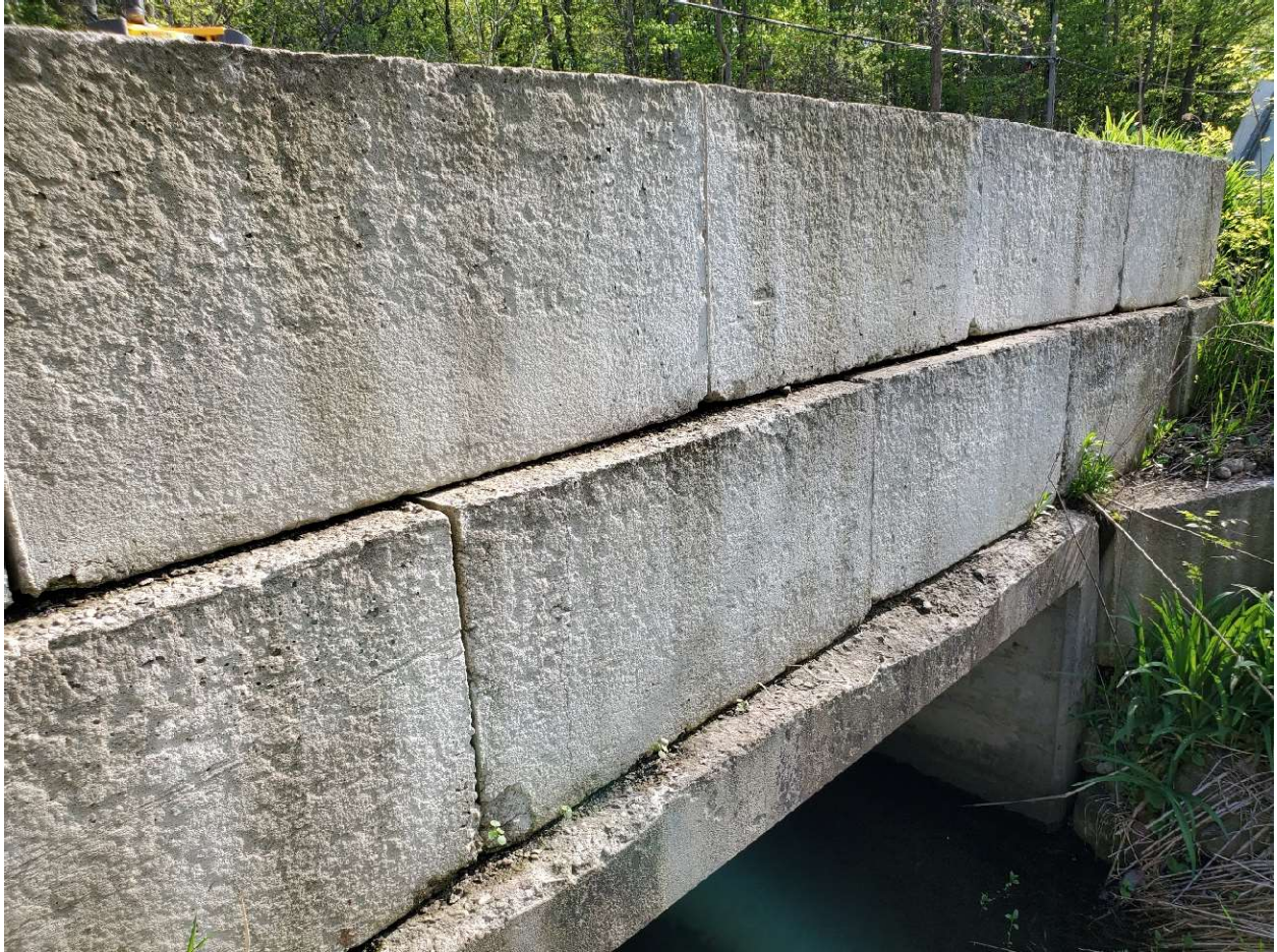
Concrete deterioration/wearing at the culvert top
