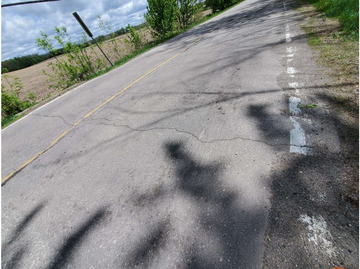
Some cracks observed in the wearing surface of the road
