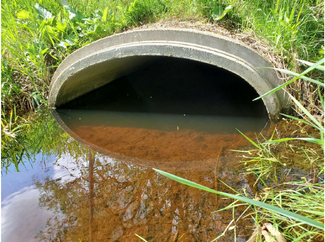
Elevation of the culvert (Some water obstruction observed)
