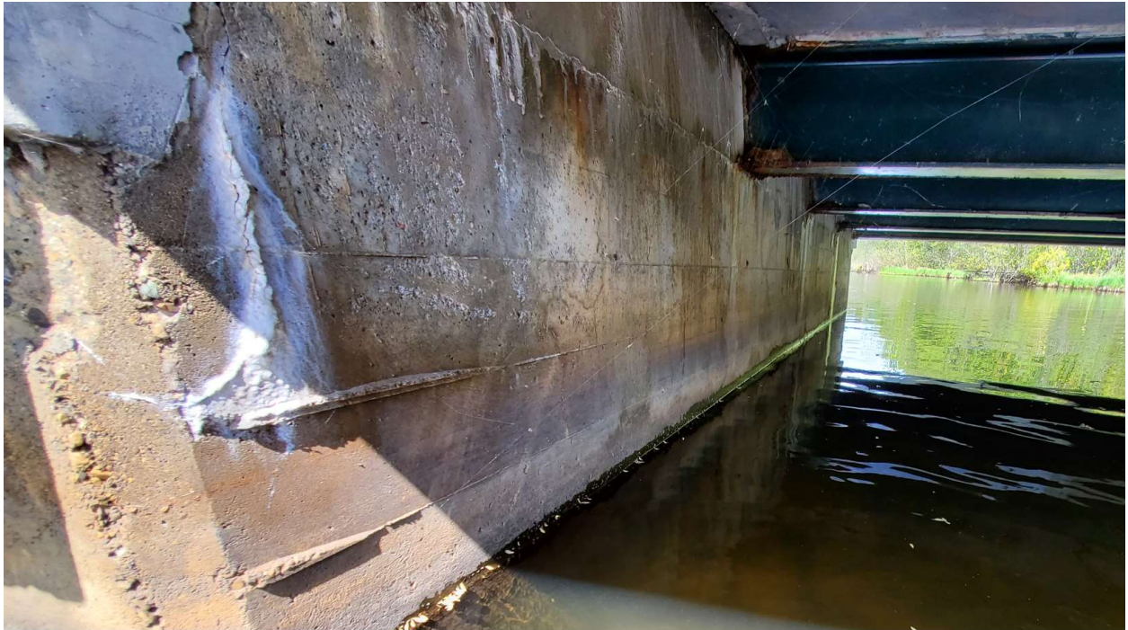
Some concrete deterioration observed at the abutment
