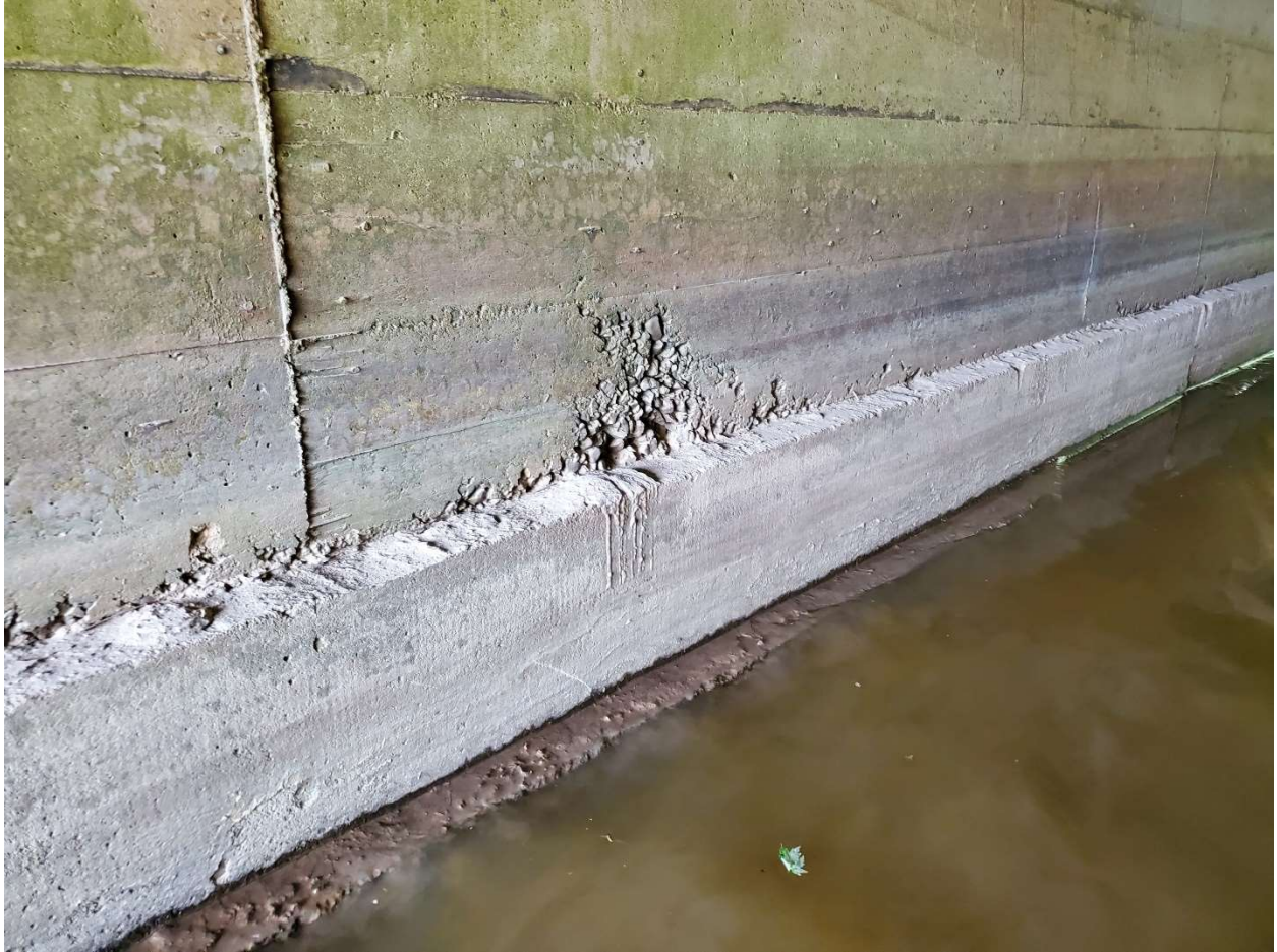
Concrete damages inside the culvert
