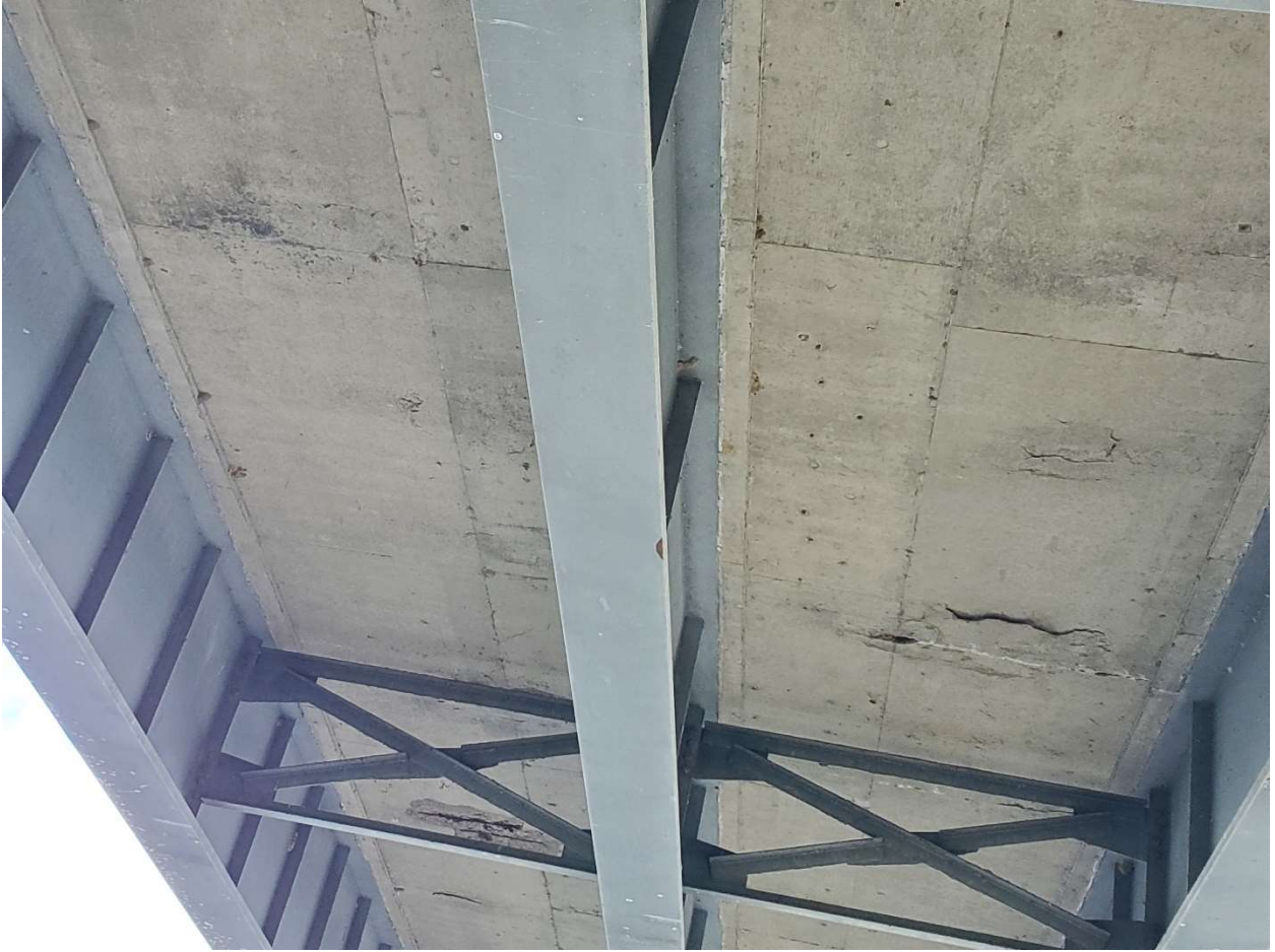
Spalling of concrete observed in Soffit
