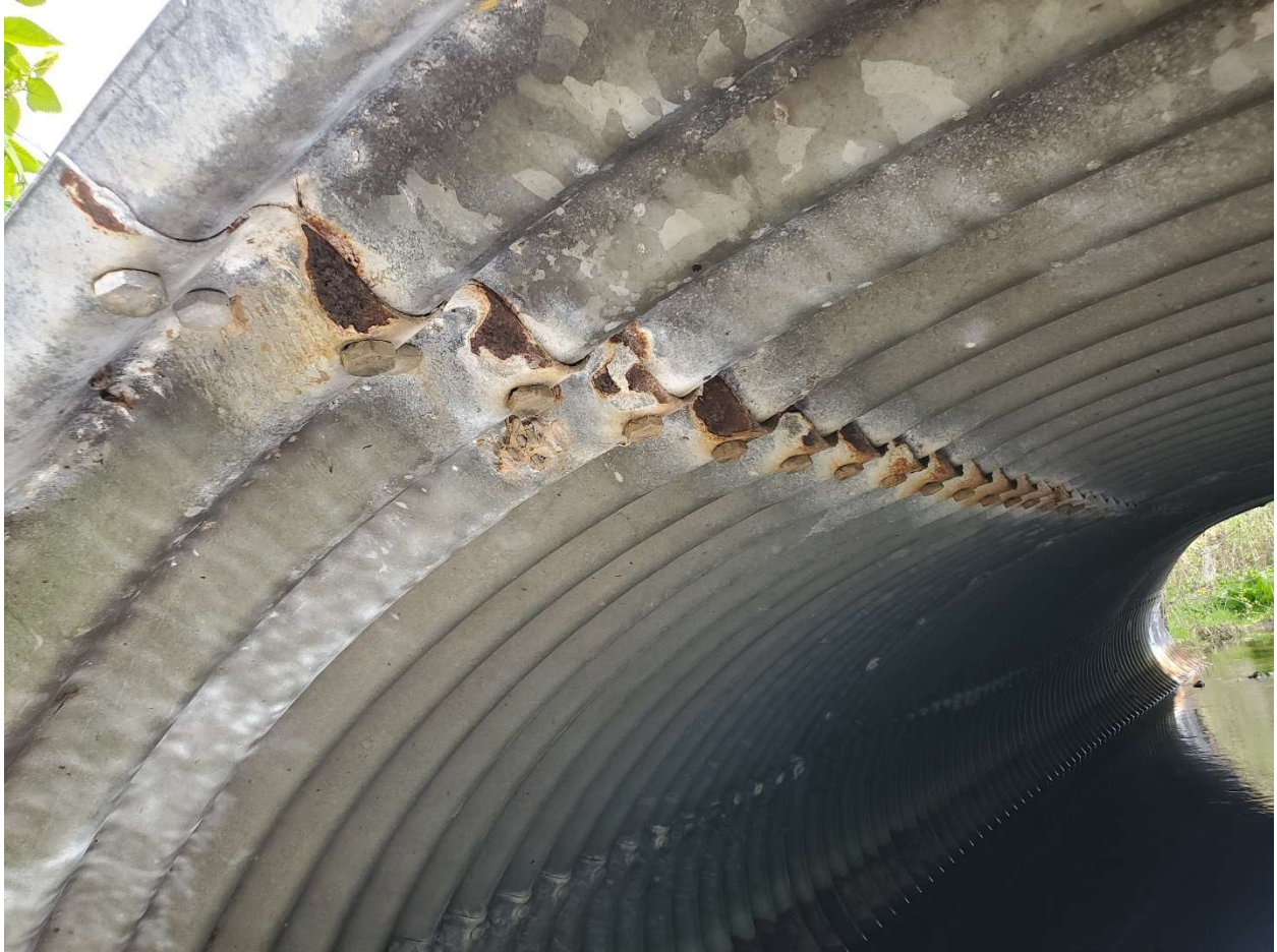
Rusting observed at Culvert joints
