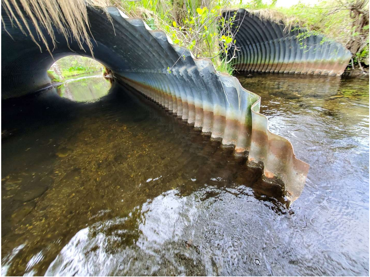
Rusting observed at Culvert bottom portion
