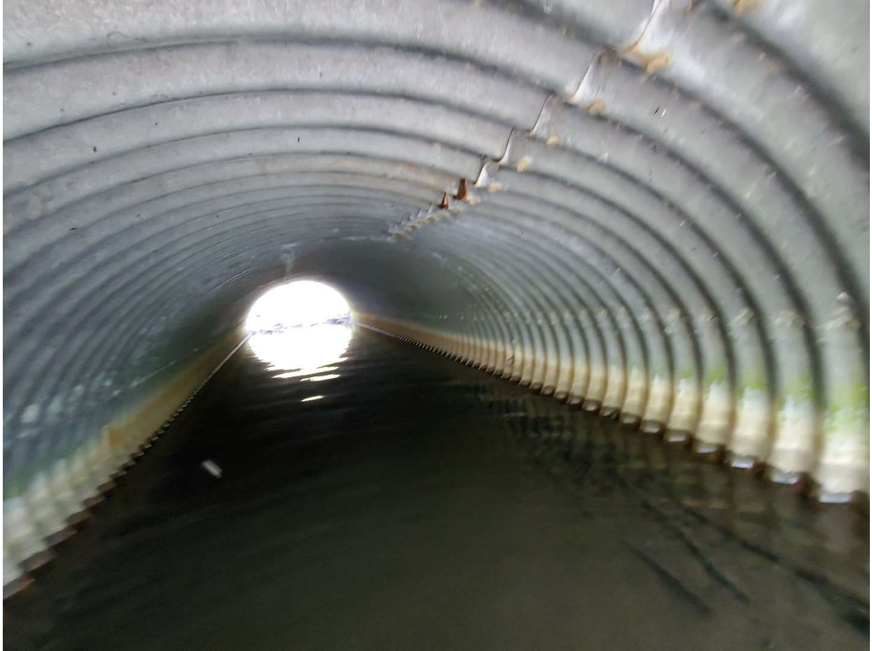
Some rusting observed at the culvert joints
