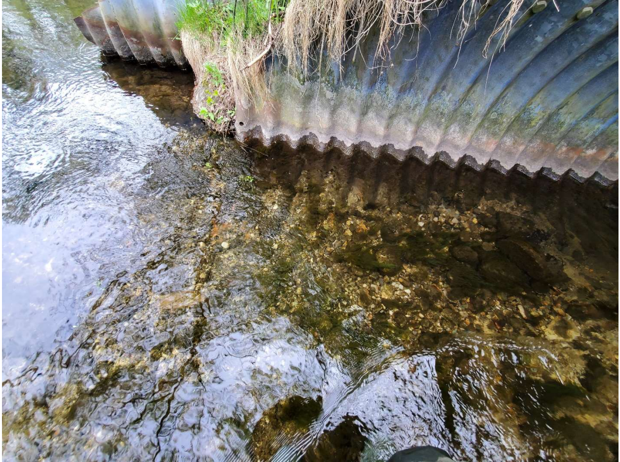
Rusting observed at Culvert bottom portion
