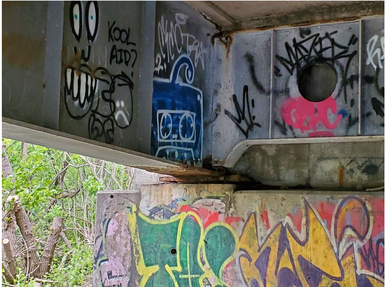
Rusting observed at the abutment
