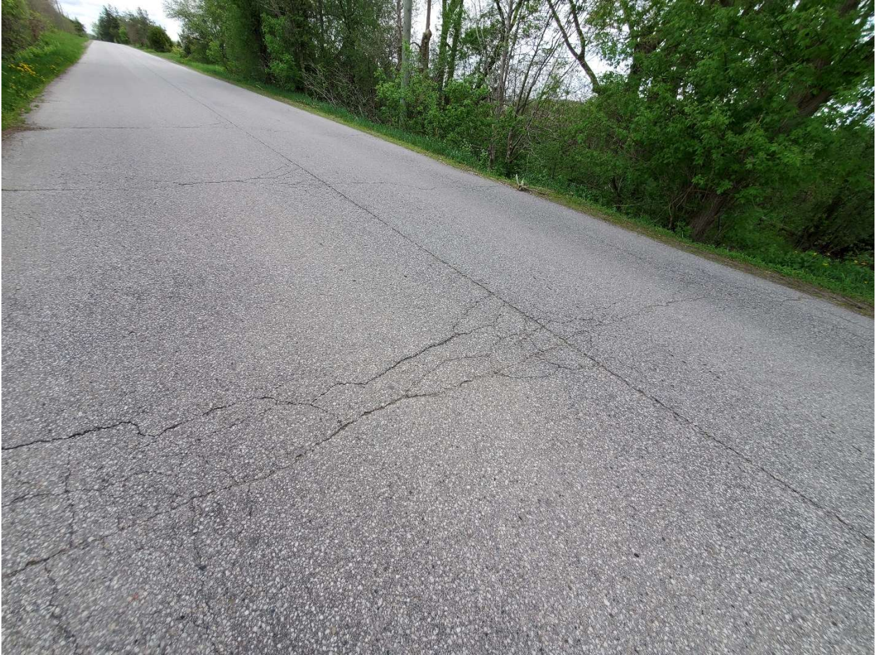
Cracks observed on the road surface
